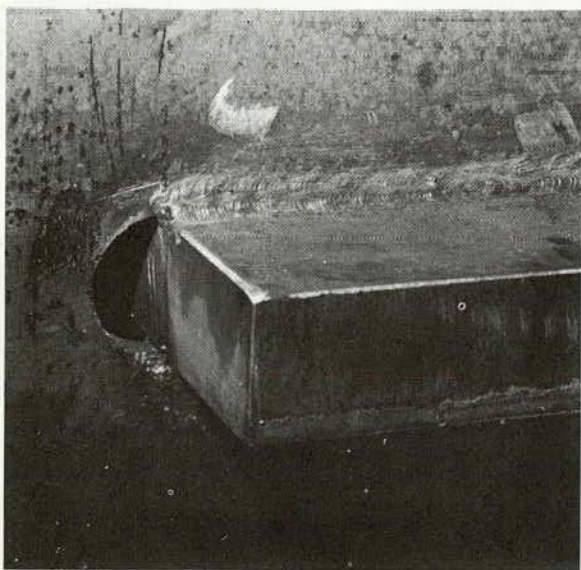
Figure 47. Coped end of flange insert.
