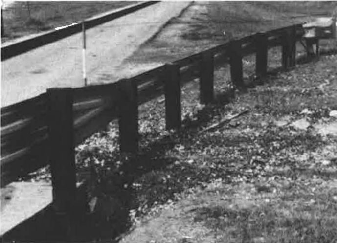
(a) Wood post installation
