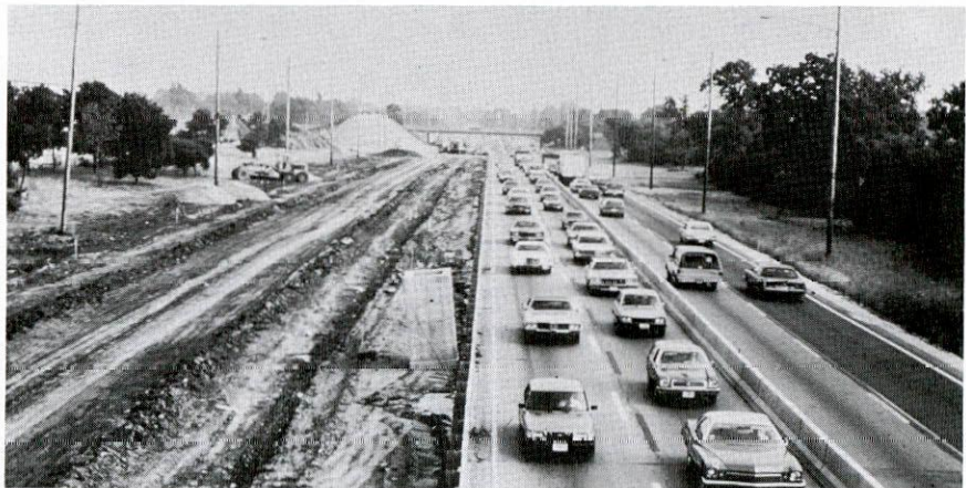
Figure 13. Reconstruction of the Eden's Expressway in Chicago used the existing three lanes and shoulder of one roadway to maintain two lanes of traffic in each direction.
