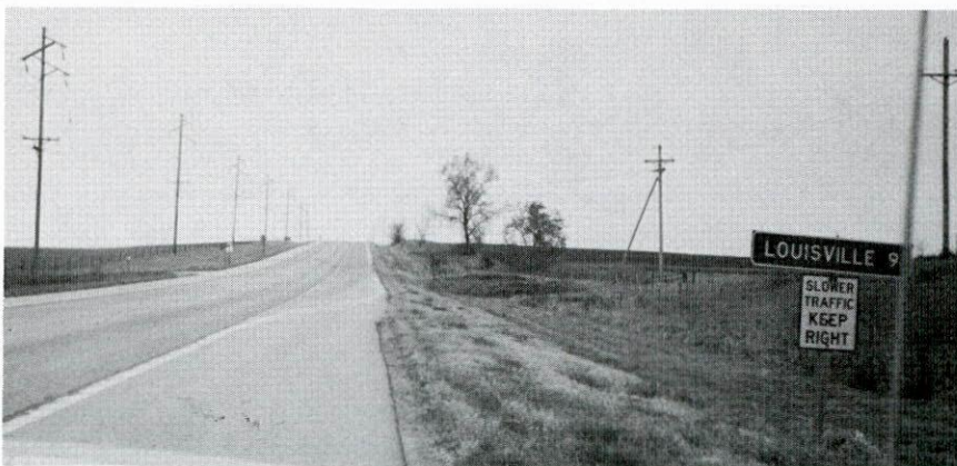
Figure 15. Paved shoulder along two-lane rural highway converted to climbing lane (note tapering of edge line stripe and advisory sign "SLOWER/TRAFFIC/KEEP/RIGHT").
