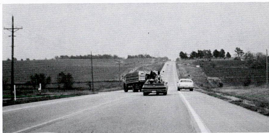
Figure 8. Paved shoulder along two-lane rural highway used by vehicle to pass truck making a left turn into driveway entrance (note edge line stripe at main-lane pavement edge).
