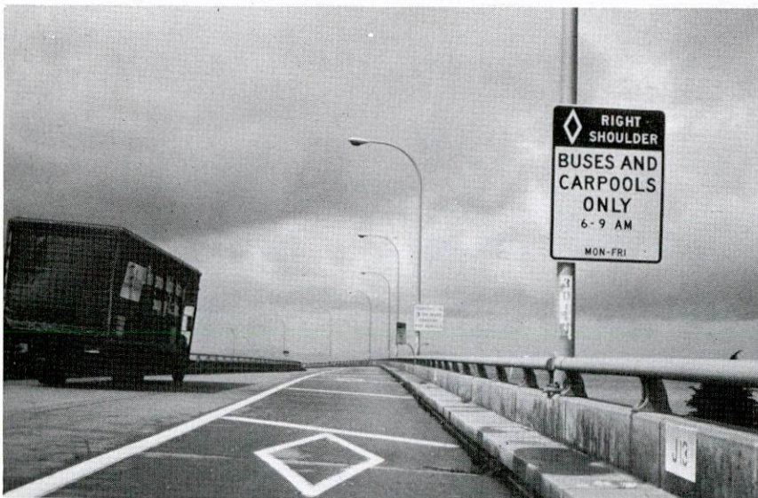
Figure 17. Use of right shoulder along elevated freeway for "Buses and Carpools Only" (note diagonal striping and diamond pavement markings).
