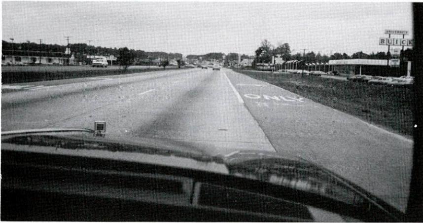
Figure 9. Paved right and left shoulders along multilane divided suburban arterial striped and marked for turns.
