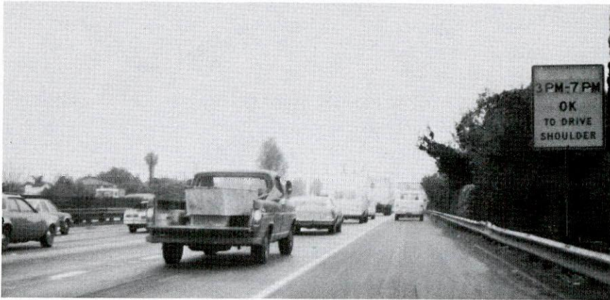
Figure 19. Permissive use of shoulder as a running lane, "3PM-7PM/OK/TO DRIVE/SHOULDER" (note normal white edge line stripe at edge of main lanes).
