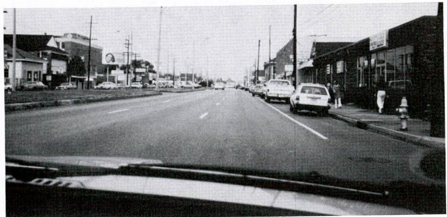
Figure 3. Eight-foot wide parking lane or parking shoulder along multilane divided city arterial street (note white edge stripe line).
