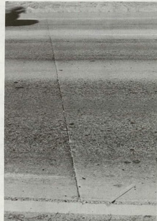
Figure 101. Studded Tire Damage (picture from jointed plain concrete pavement).
