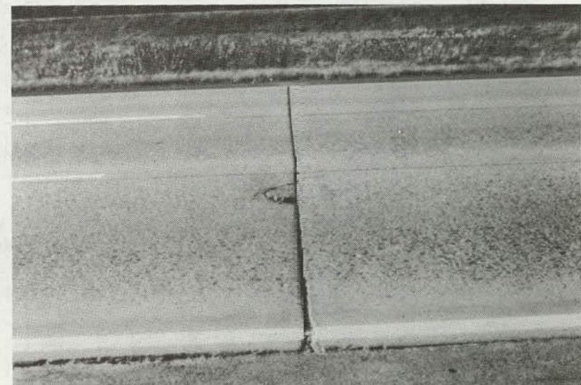
Figure 93. Low-Severity Spalling.
