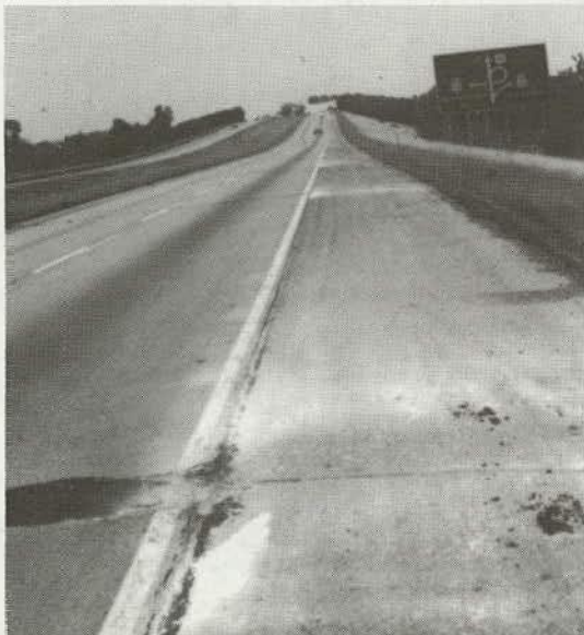
Figure 88. High-Severity Pumping.
