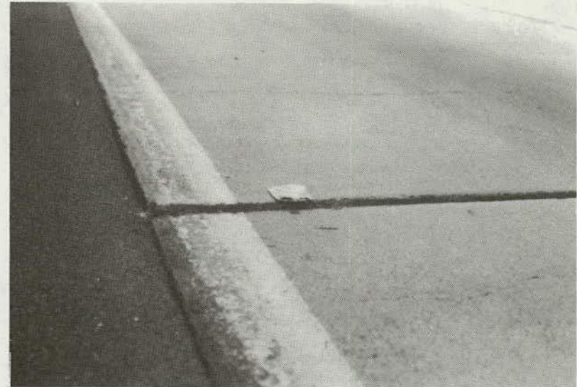
Figure 68. Joint Faulting.
