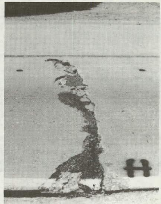
Figure 96. High-Severity Spalling.
