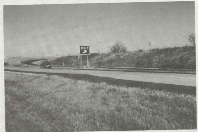
Figure 161. Swell Caused by Expansive Soil.
