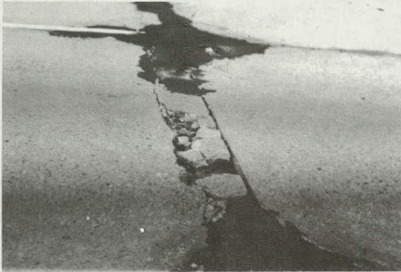
Figure 100. High-Severity Spalling.
