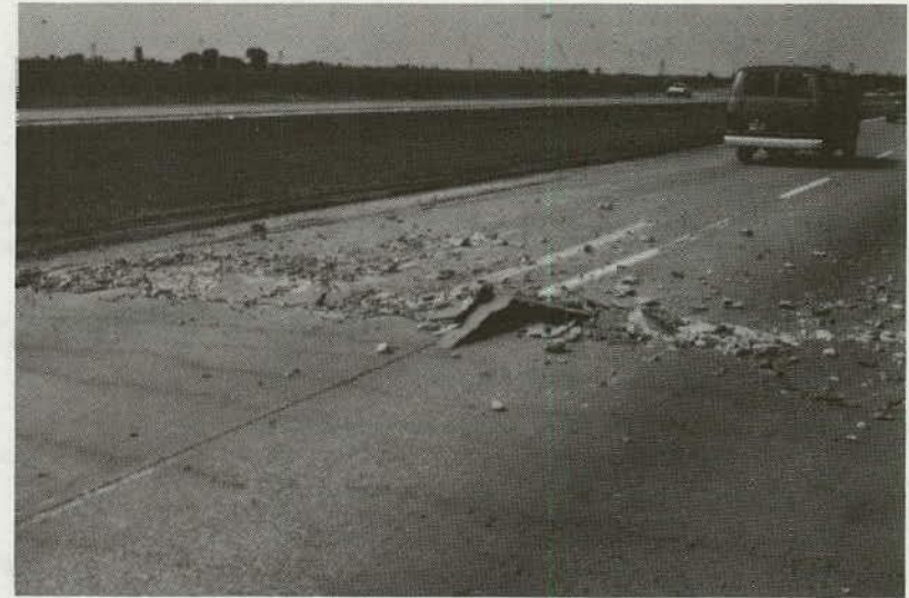
Figure 109. High-Severity Blow-up.
