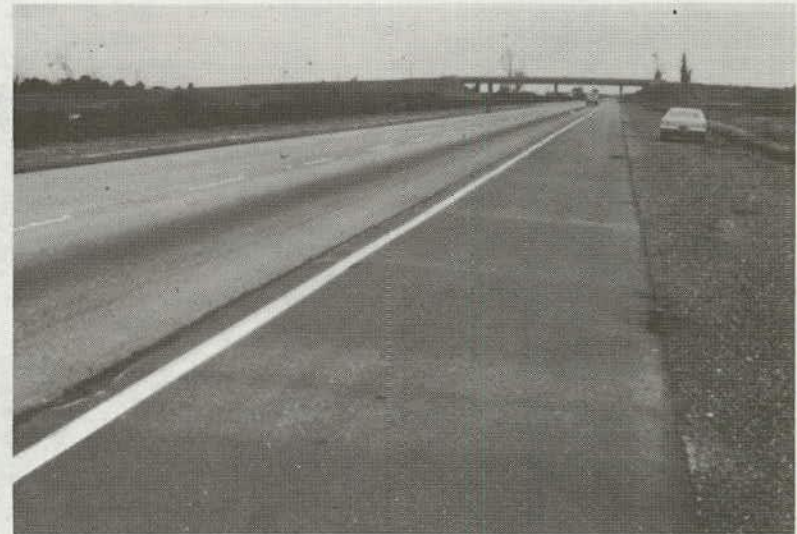
Figure 35. Medium-Severity Pumping.
