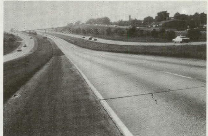
Figure 18. Joint Faulting.
