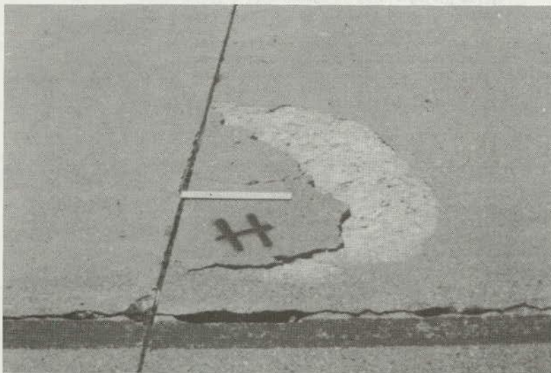
Figure 95. High-Severity Spalling.
