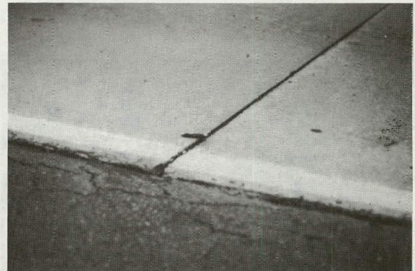
Figure 18. Joint Faulting.
