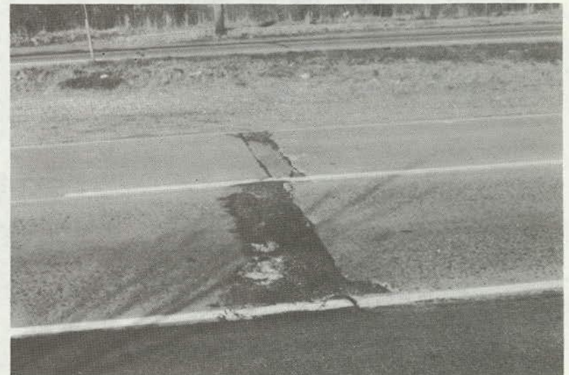
Figure 99. High-Severity Spalling.
