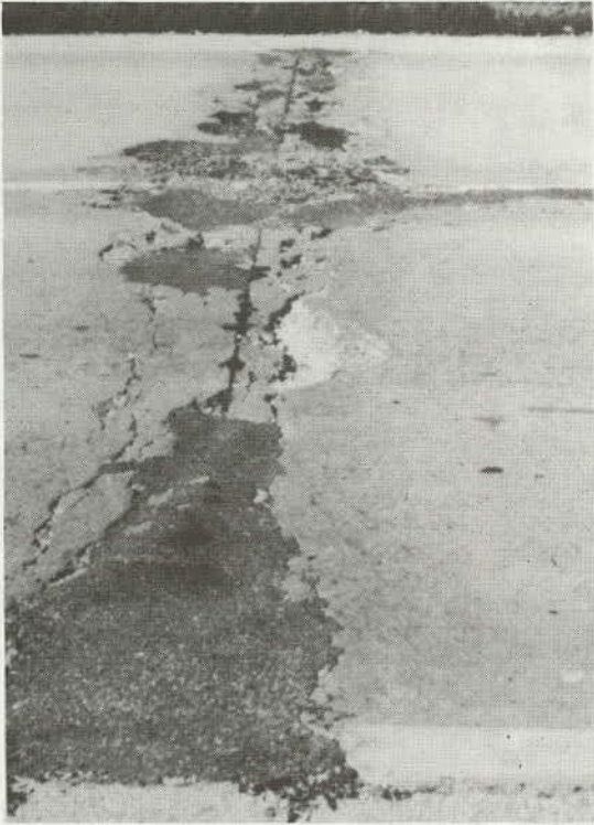
Figure 97. High-Severity Spalling.
