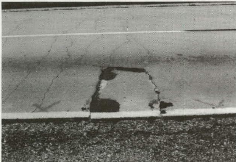
Figure 120. Medium-Severity Edge Punchout.
