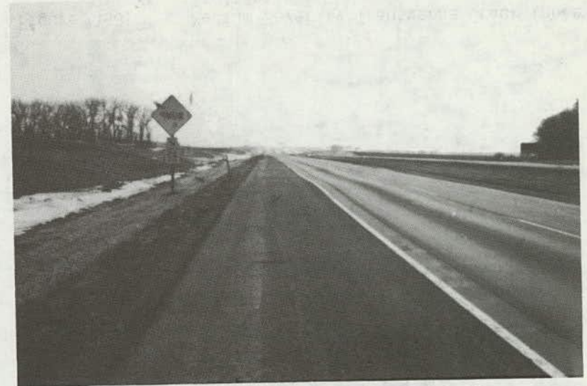
Figure 160. Swell Caused by Frost Heave.
