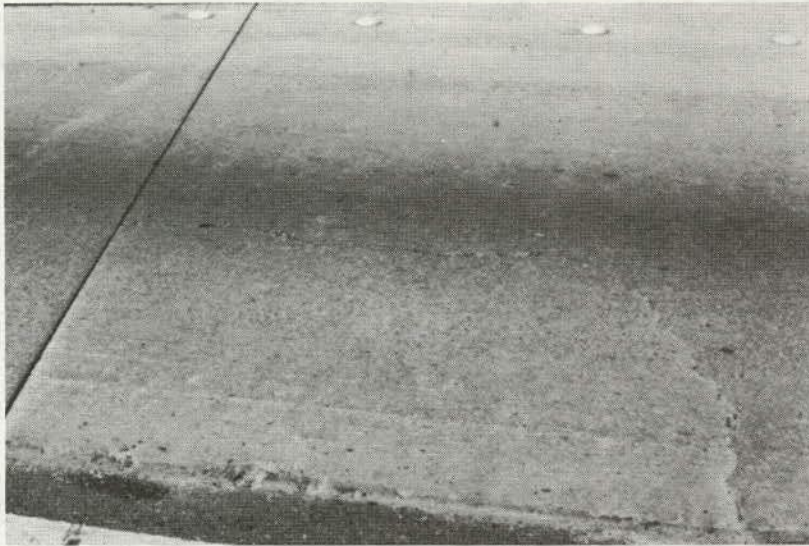
Figure 12. Corner Break.
