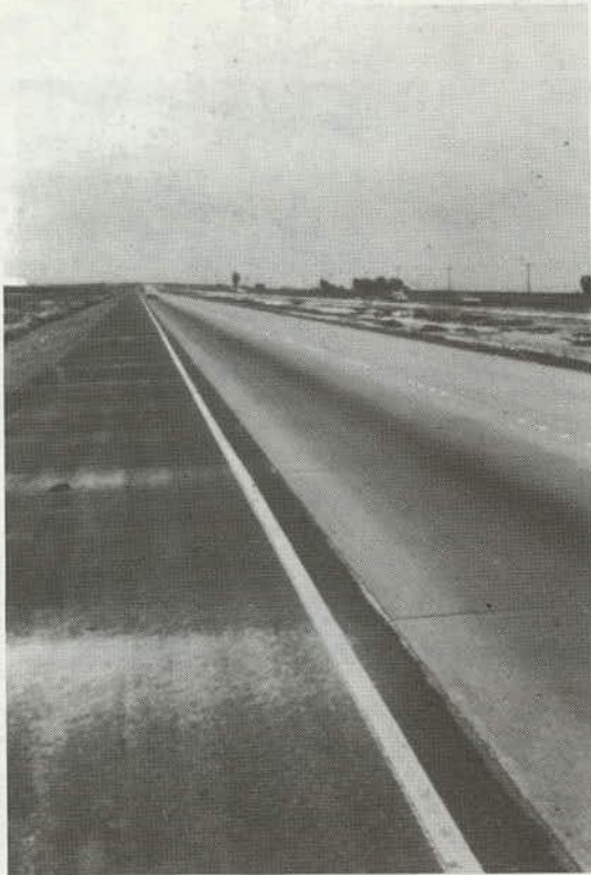
Figure 36. High-Severity Pumping.
