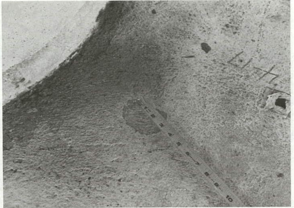
Figure E-2. Small scaled areas on top of the base.
