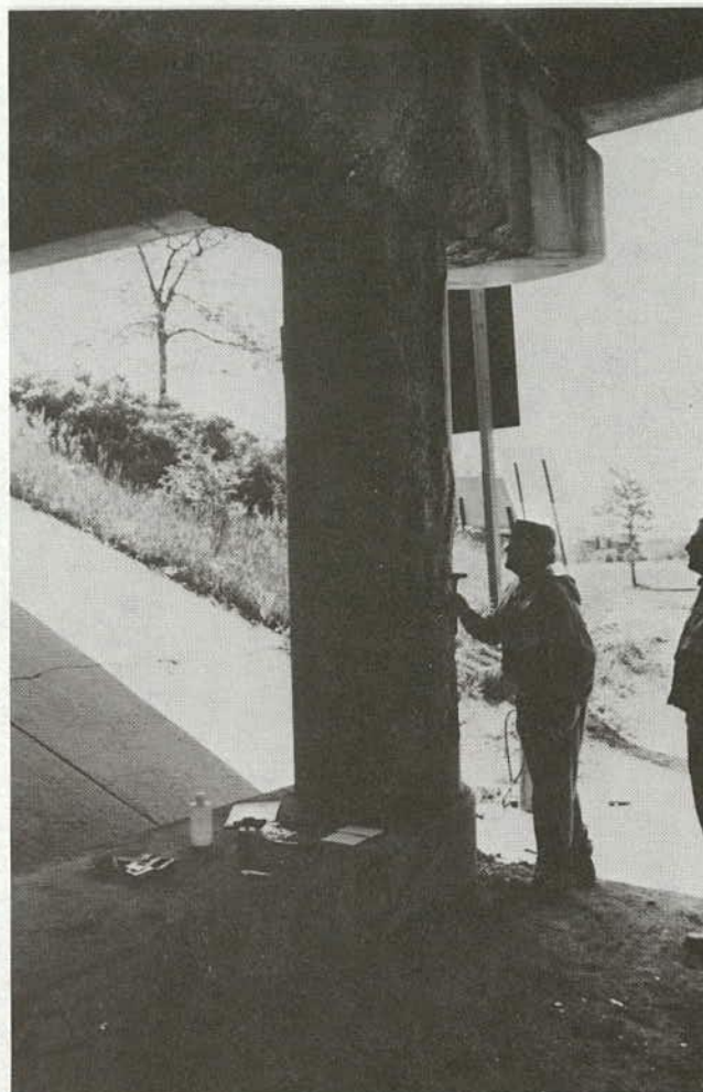
Figure C-1. General deterioration of pier base, column and cap (south end).
