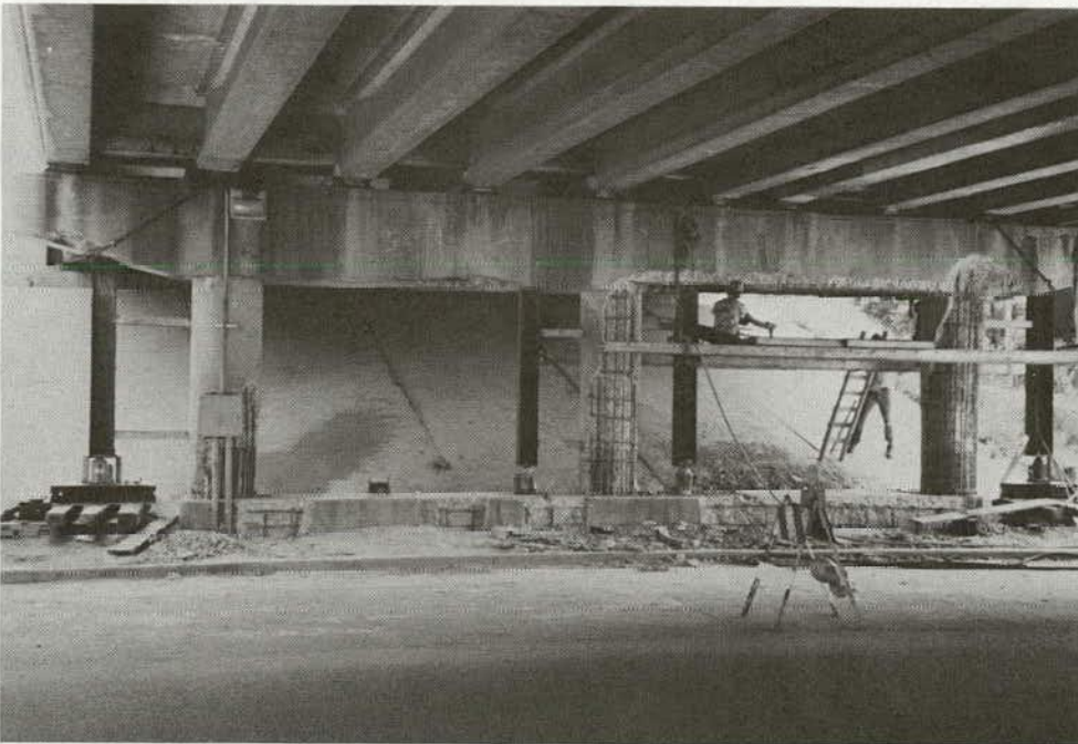
Figure C-4. Bridge pier after removal of majority of delaminated and unsound concrete.
