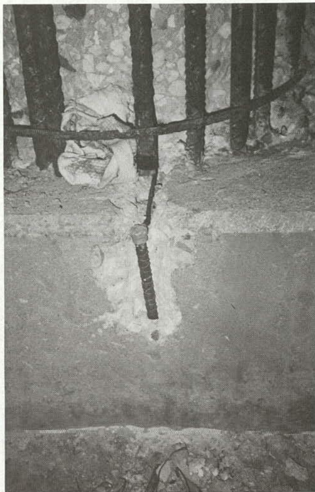
Figure C-9. Rebar current pickup probe in place.
