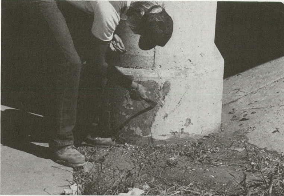
A. Scraping coating off a scaled area of the base.
