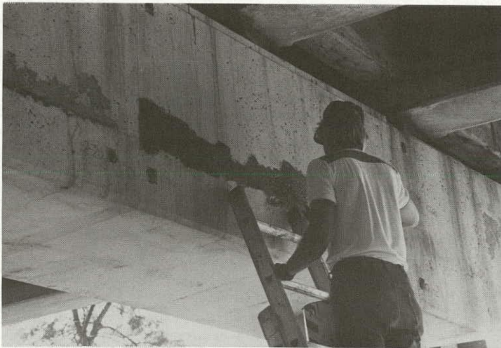
Figure E-4. The largest areas of scaled conductive coating.
