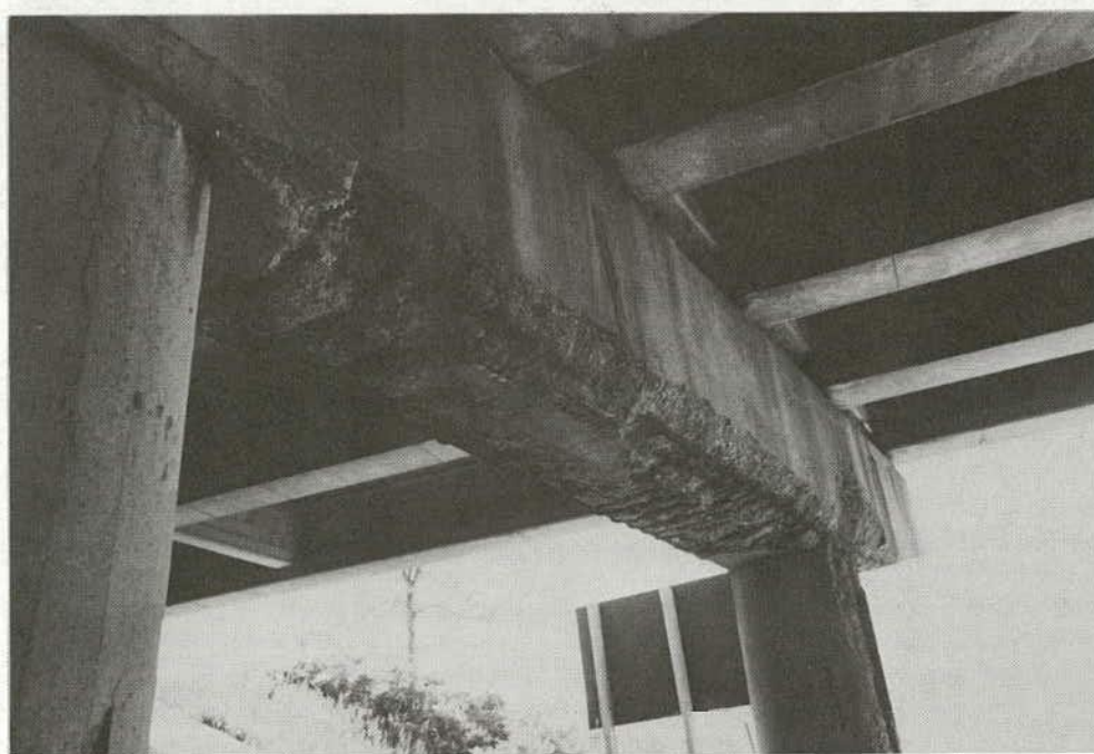
Figure C-1. General deterioration of pier base, column and cap (south end).
