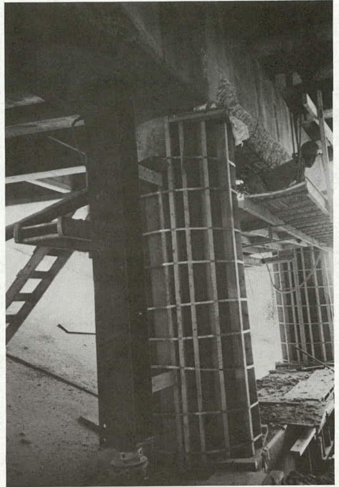
Figure C-5. Wood form details for column repair.
