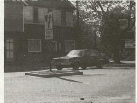
(c) The triangular traffic island in the middle of the intersection serves no channelization function.
