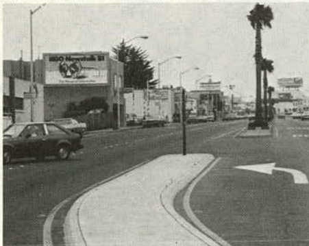
(d) Exclusive u-turn channelization just north of Como Avenue serves southbound traffic from Gambetta and Como.
