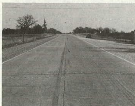
d) and e) The long taper develops a left turn lane for west to north movements.
