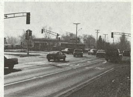
(c) Large radius and wide throat provide for good operation of double left.
