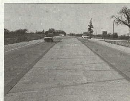
c. Painted channelization provides separation of opposing flows, protection for the west to north left turn lane, and visual notice of the intersection.
