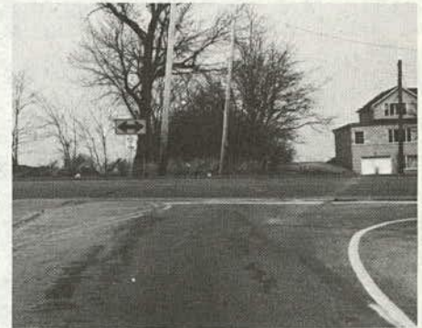
(f) The stopped approach on Quentin Road is separated from opposing volumes by a painted island.
