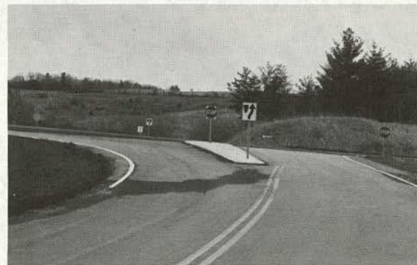
Channelization should clearly separate opposing traffic flows.
