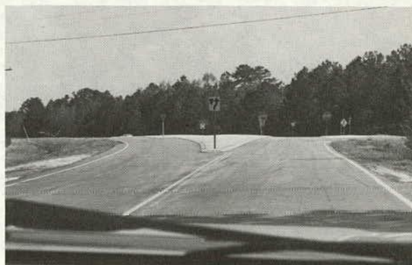
Approach noses to median islands should be offset from the traffic lanes.
