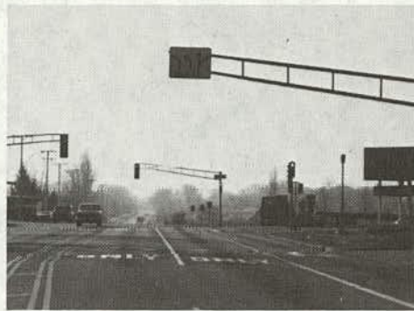
(a) and (b) Pavement markings and overhead signaling are provided well in advance of the intersection to alert approaching drivers.
