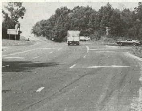
(d) The more compact, conventional intersection form provides clear sight lines, small conflict areas, and understandable operation for all drivers.
