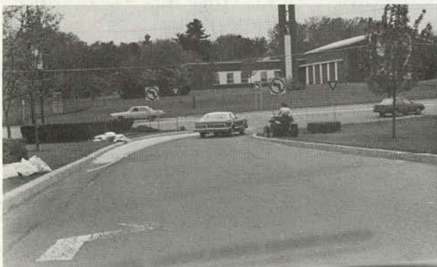
Driveway design encourages the right turn only movements
