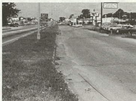
(b) The "normal" frontage road/Mastin Street cross section is shown here. Note the land use along the frontage road.
