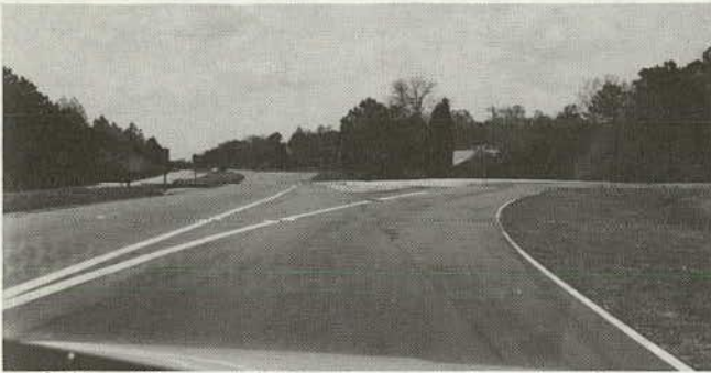
A full offset and blunt approach end radius are appropriate for traffic islands at high-speed right turn lanes.
