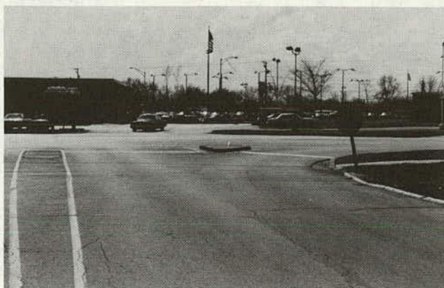
This triangular island is too small to serve any channelization function.
