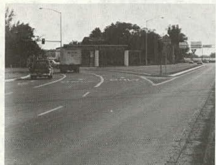
(d) Through traffic onto Exposition Drive proceeds on a smooth, flat horizontal curve. Note the blunt approach end of the "right" turn lane island nose.
