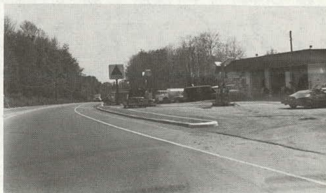
Right turn lanes remove rear-end conflicts in advance of crossing conflicts at unsignalized intersections.
