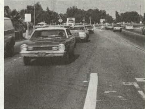
(b) The short left-turn lane from State Route 178 was frequently blocked by queues.
