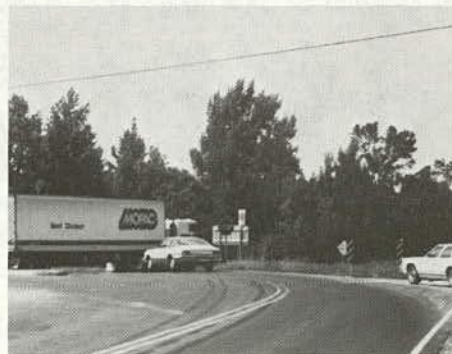
(e) The U.S. Route 1A approach leg is realigned to create an angle of intersection closer to 90°.
