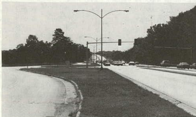
Separation between frontage roads and through arterials eases the driver's task of handling multiple conflicts.
