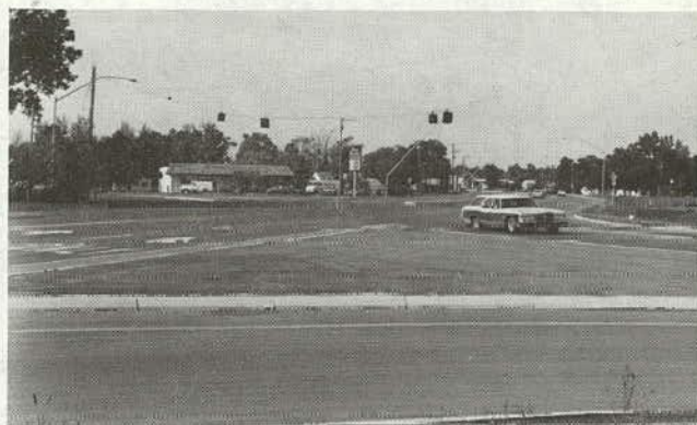
Right turn lanes remove rear-end conflicts in advance of crossing conflicts at unsignalized intersections.
