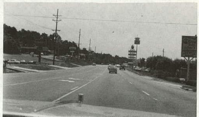
Continuous two-way left turn lanes promote safe access to multiple drive-ways outside higher speed through lanes.
