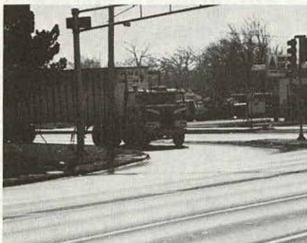
(d) and (e) Right turn roadway width and radius design enable easy turns by frequent semi-trailers.
