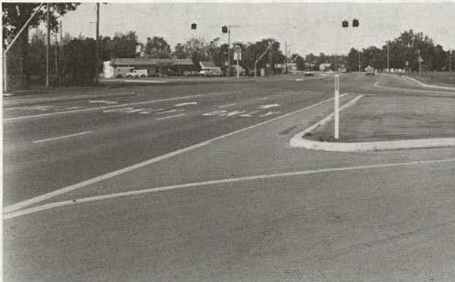
Good offsets on this approach end promote safe operation of the high speed turning roadway.
