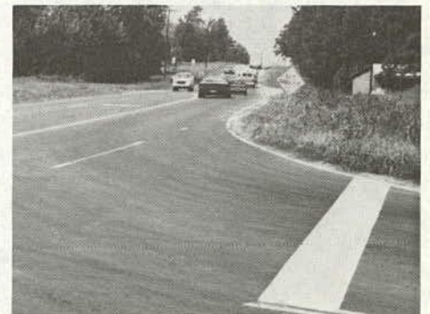
(f) Right turns from U.S. Route 1A are aided by an 80-foot radius return.
