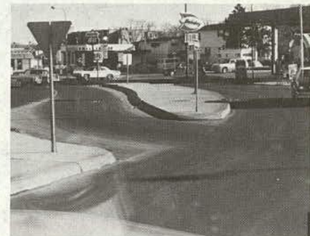
(c) Design of the channelization provides protection for stopped vehicles, clearly defines the through route, and produces conflict angles of about 90°.
