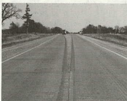
d) and e) The long taper develops a left turn lane for west to north movements.
