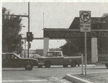
(f) The 90° angle of intersection produces a compact intersection with small conflict areas. Note the small right corner radius, which discourages undesirable right turns.
