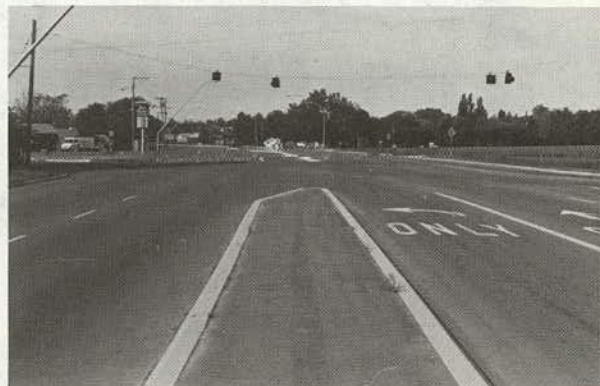
Tapers that are too short appear "stiff" and unnatural, and are not consistent with vehicle paths.
