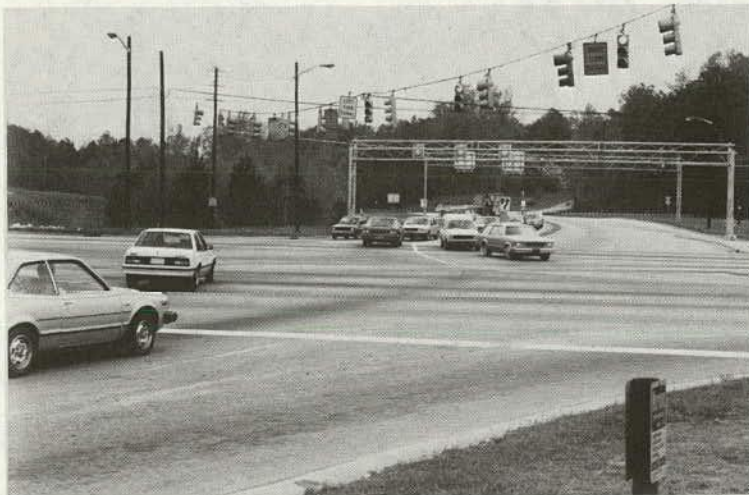
Good design promotes simultaneous discharge from both lanes.
