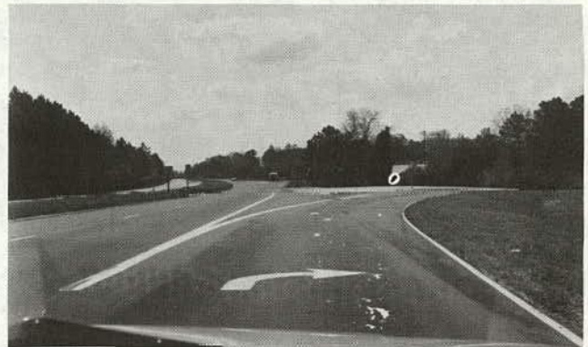
Right turn deceleration lanes off high-speed highways promote safe turning speeds.
