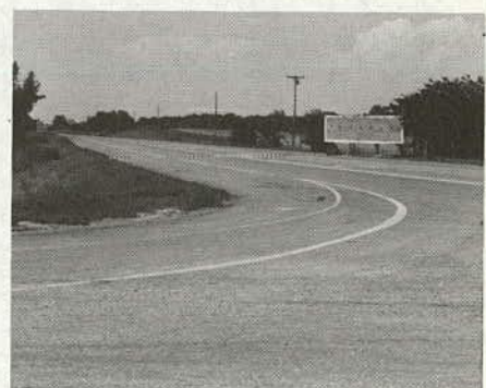
(f) Note the 75-foot radius return and sight distance from the stopped approach on U.S. 24.
