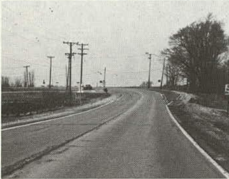
(a), (b) and (c) The bypass lane for westbound traffic begins about 300 feet in advance of the intersection. It is intended for optional use by through drivers who encounter queued left turning vehicles in the left lane. The bypass lane merges back into the through lane past the intersection.
