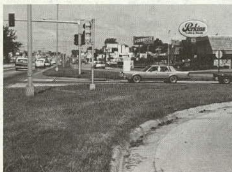
(a) The frontage road is relocated away from 63rd Street to provide separation between frontage Road/Mastin Street conflicts and the 63rd Street signalized intersection. Storage for about 3 passenger cars is created.
