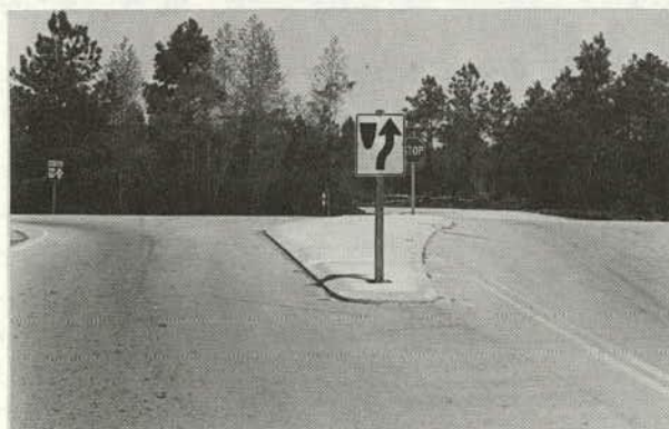
Approach noses to median islands should be offset from the traffic lanes.
