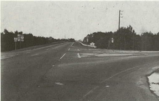
Note the continuous tapering effect created by careful placement of both corner islands.
