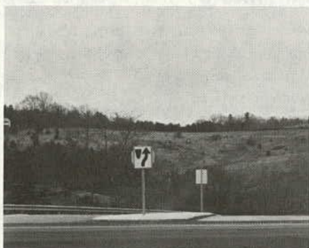
(c) and (d) Raised median channelization is effective in guiding vehicles across the intersection.
