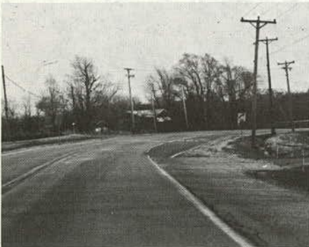
(d) and (e) An exclusive right turn lane provides for safe deceleration for the heavy right turn volume from Old McHenry Road. Clear sight lines to the cross road are evident from the photo at right.
