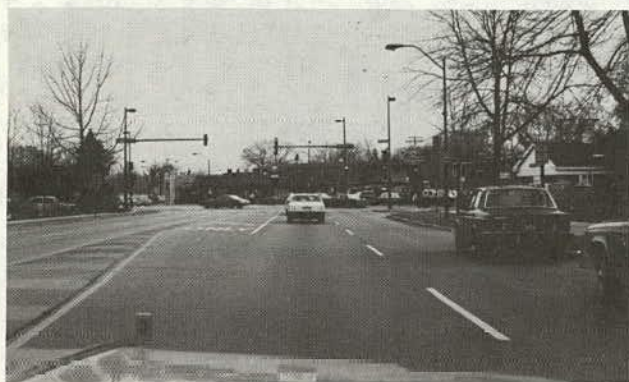
Left turn lanes facilitate signal phasing.
