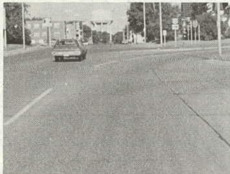
(a) Before construction, eastbound traffic on U.S. Route 10 encountered large open pavement, with no protection for vehicles bound for Frazee Street. The continuity of U.S. Route 10 is not clearly defined.
