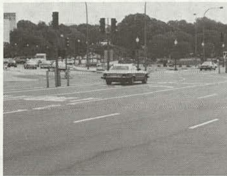
(a) and (b) Well-marked double left turn lanes and turn Constitution Avenue traffic into a 36-foot throat.
