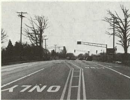
(a) and (b) Pavement markings and overhead signaling are provided well in advance of the intersection to alert approaching drivers.
