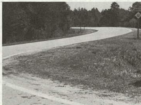
(b) and (c) The new alignment provides good sight angles to both legs for drivers at the stop line. Note the cleared roadsides which provide sufficient corner sight distance.
