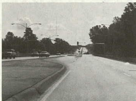
(d) The left turn lane to Mastin Street is contained within the raised median. The channelization allows for unstopped eastbound movements along 63rd Street.
