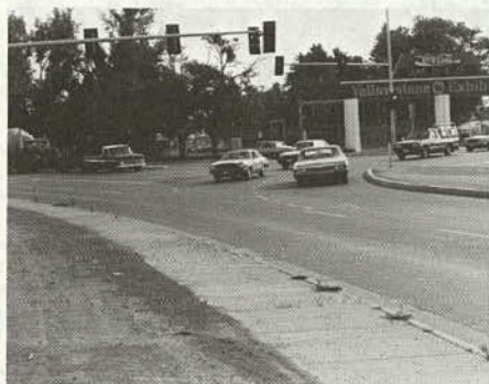
(a) Auxiliary pavement markings and a wide throat assist the movement of the double left turn from the east leg.
