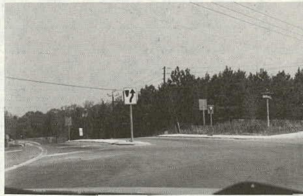
Traffic islands physically separate opposing traffic flows.
