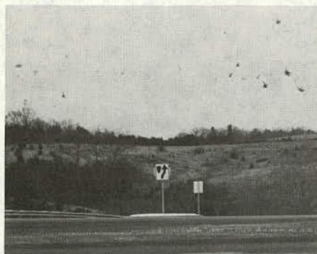
(c) and (d) Raised median channelization is effective in guiding vehicles across the intersection.
