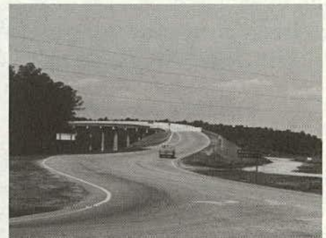
(b) and (c) The new alignment provides good sight angles to both legs for drivers at the stop line. Note the cleared roadsides which provide sufficient corner sight distance.
