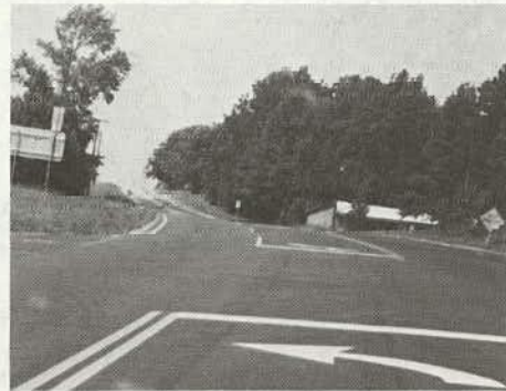
(a) and (b) Fully shadowed left turn lanes are provided with painted approach tapers. The long approaches give good advance notice of the intersection past the mild horizontal curve.
