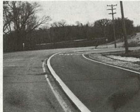
(d) and (e) An exclusive right turn lane provides for safe deceleration for the heavy right turn volume from Old McHenry Road. Clear sight lines to the cross road are evident from the photo at right.
