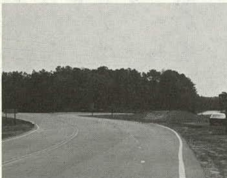
(d) and (e) A right turn lane is provided for eastbound U.S. Route 70 vehicles. Note the smooth taper. Also note the full lane offset of the median island nose.
