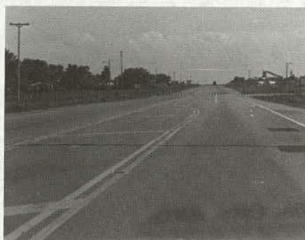
(b) and (c) The design of the left turn lane requires turning vehicles to make a positive maneuver into the lane. Pavement arrows confirm the lane designation.
