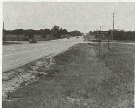
(d) Excellent sight distance is available in all quadrants of the intersection. All signs were relocated inside a 1500-foot sight line on the approaches to U.S. Route 24.
