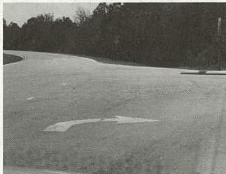
(d) and (e) A right turn lane is provided for eastbound U.S. Route 70 vehicles. Note the smooth taper. Also note the full lane offset of the median island nose.
