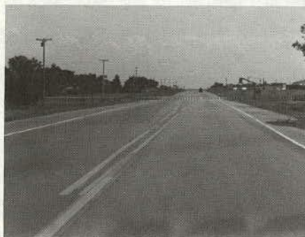
(a) The approach taper for the left turn lane and excellent sight lines provide clear notice of the intersection to through drivers on U.S. 81.
