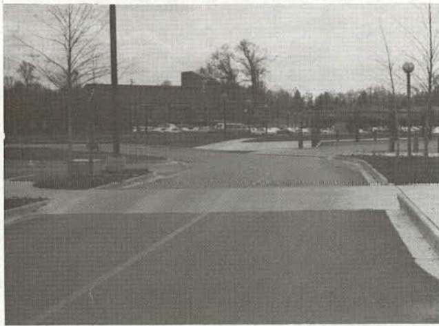
Figure 31. Elevated walkway/speed hump. (These elevated walkways at the Brandermill PUD provide a convenient path for pedestrians while controlling vehicle speeds. However, they are underused.)
