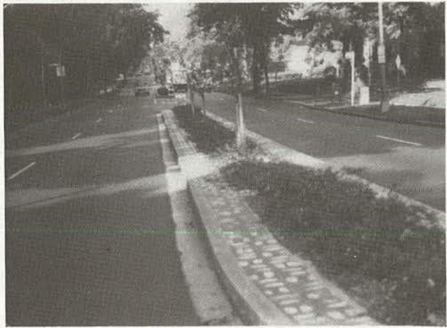
Figure 74. Retrofitted median on 16th Street in suburban Washington, D.C.
