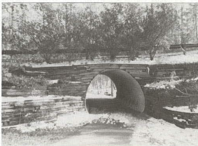
Figure 26. Inexpensive pedestrian/bicycle underpass provided in Brandermill.
