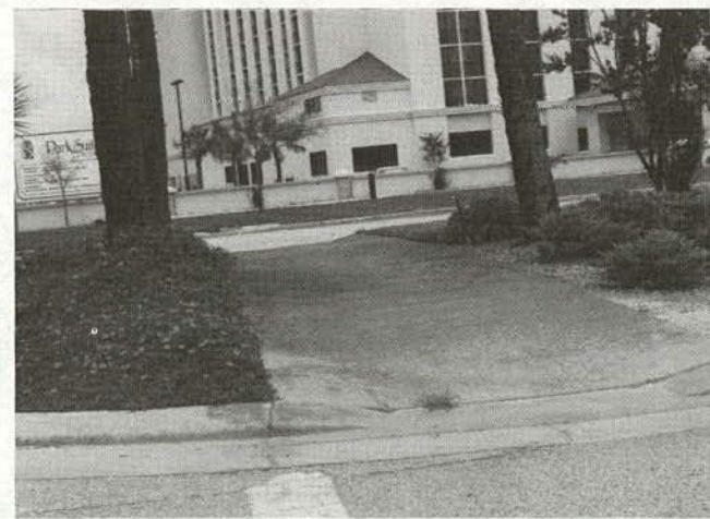
Figure 70. Well-designed-elevated median crossing.
