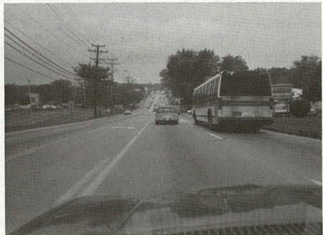
Figure 5. Arterial highway with a two-way left-turn lane.
