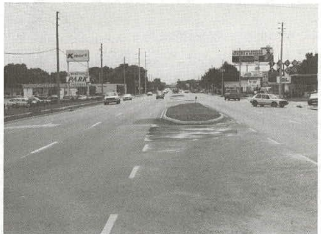
Figure 67. Application of short median segments to a wide arterial street.
