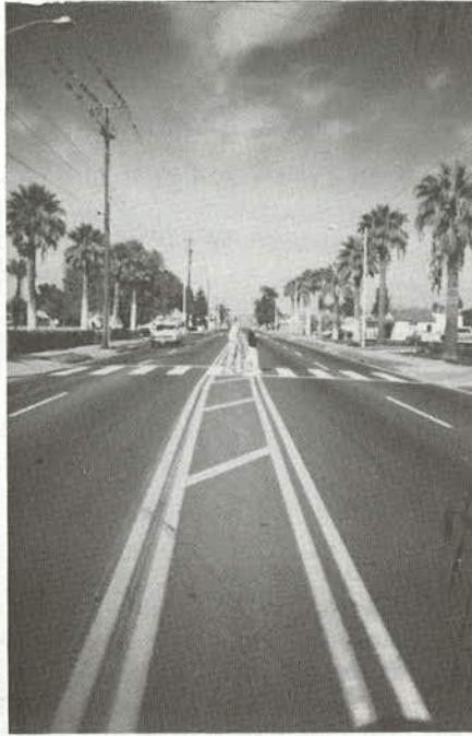
Figure 75. Retrofitted striped median in Phoenix to solve a pedestrian crossing problem.
