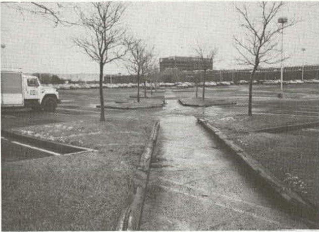
Figure 29. Diagonal pathway through parking lot constructed using islands at each parking aisle.
