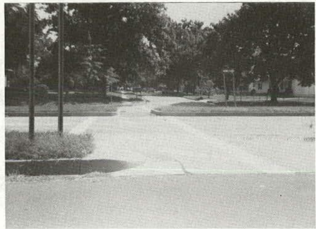
Figure 69. Median opening to accommodate street-level pedestrian crossings.
