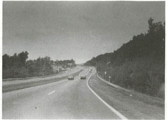
Figure 71. High-speed suburban arterial with 10-ft paved shoulder.
