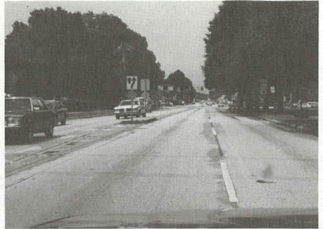
Figure 78. Pedestrian refuge island linking a parking lot and office in Orlando.
