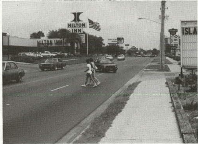
Figure 18. Example of inconsistencies in sidewalk setback (see right side of photo).
