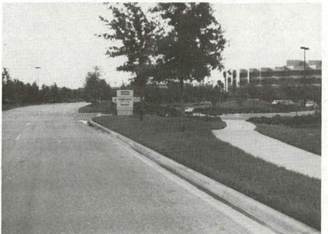
Figure 73. Variable walkway separation to accommodate meandering paths.
