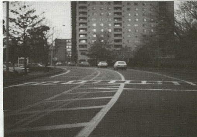
A bold, painted median can give the pedestrian some refuge, but a raised median or refuge island would be much better.
