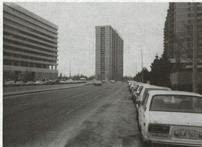
South George Mason Drive. Note construction of pedestrian bridge in the distance.
