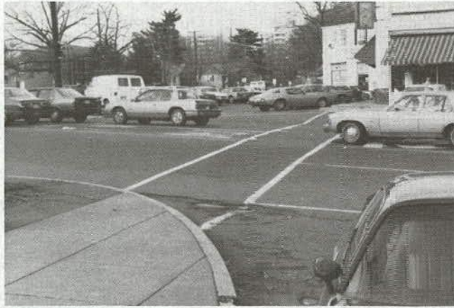
Where the major crossing point is not at the intersection itself, an auxiliary crosswalk may be needed to delineate the crossing area and to discourage vehicles from blocking it.
