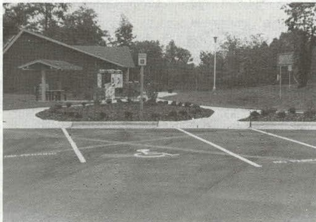
Parking lots should be striped to prohibit vehicle parking where walkways enter the parking lot.
