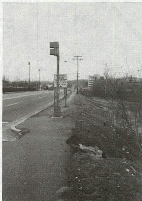
Sidewalk from Amtrak parking area to the crossing of Garden City Drive. Note worn path up the east side of Garden City Drive.
