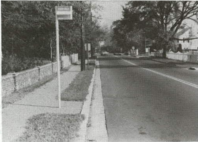
Paving across the planting strip at bus stops provides a stable, mud-free surface for pedestrians.
