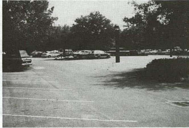
Well-landscaped and channelized parking lot. Islands control traffic but allow for ease of pedestrian movement diagonally toward shopping center.
