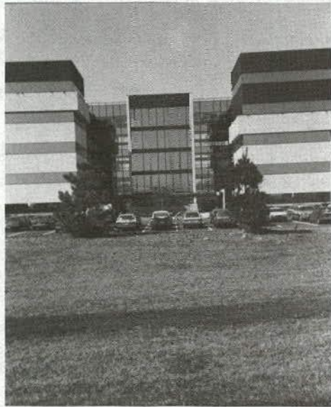
View from sidewalk to building entrance. You can not get there from here.
