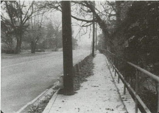
Where guardrail is needed at embankments, it is preferable to place the pedestrian walkway outside the guardrail .
