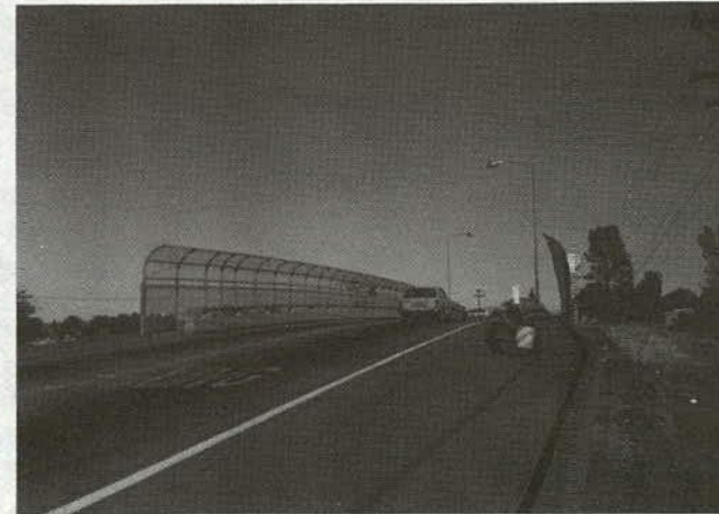
Protective barriers for pedestrians at bridges are also a positive feature, and need not be expensive. However, the end treatments are important for vehicle safety.
