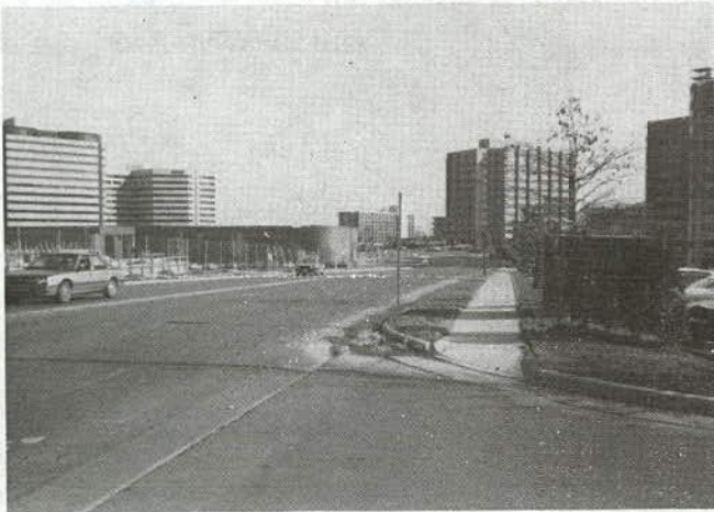
Sidewalks are being provided in some of the newer areas. A median or refuge island would have helped the pedestrian crossing situation here.
