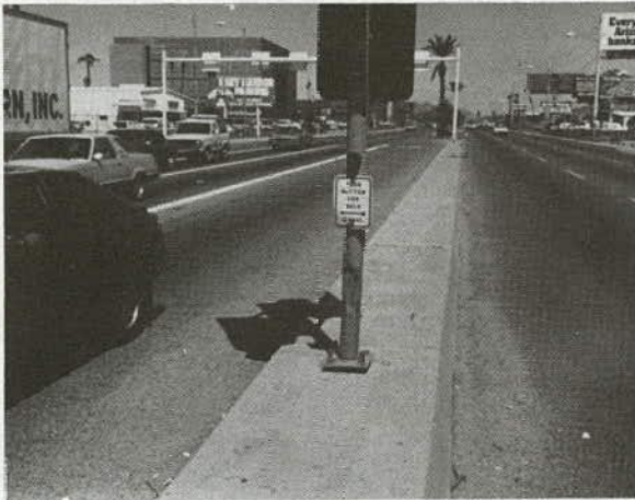
Pedestrian push buttons on the median can assist stranded pedestrians.
