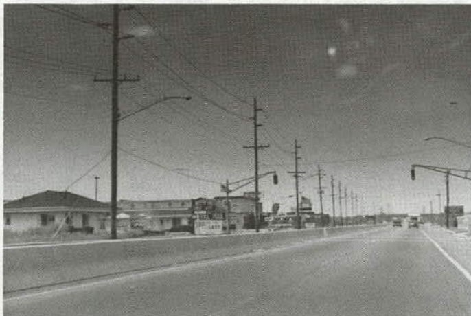
The pedestrian crossing signal and opening in the barrier are provided for access between two commercial establishments on this arterial.
