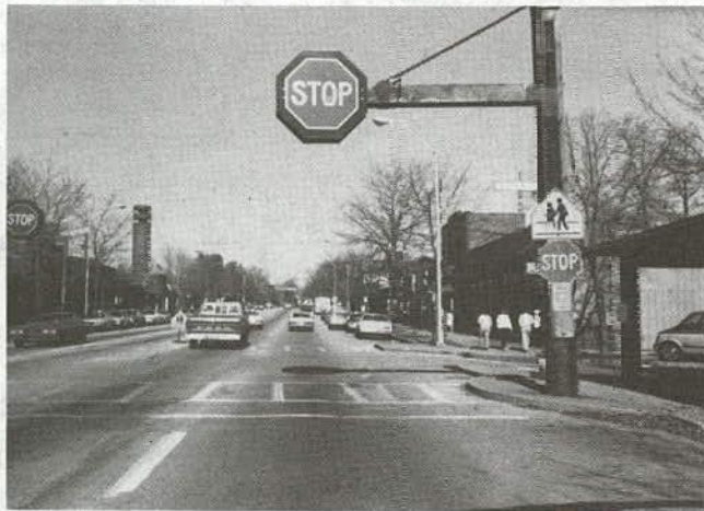
Unique crossing treatments can be provided where vehicles enter a predominately pedestrian precinct. They can also add to the area's character.
