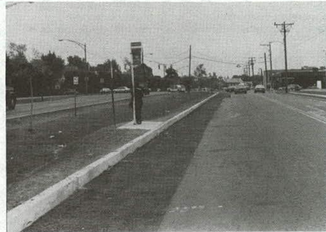
Small concrete pads for bus stops a simple but welcome addition. This one required only a slight widening of the embankment.
