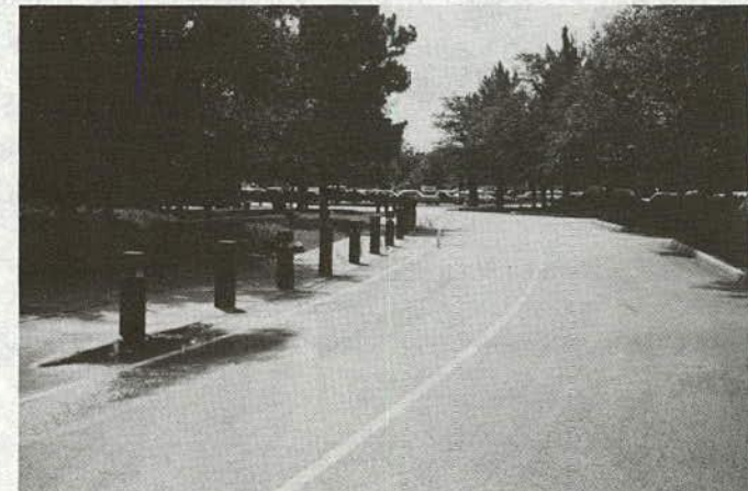
Roadway adjacent to shopping center. Note street-level sidewalk separated from road by bollards and pedestrian level lighting.
