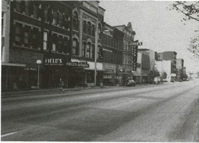
Looking north on Main Street. Note extended sections of curb.
