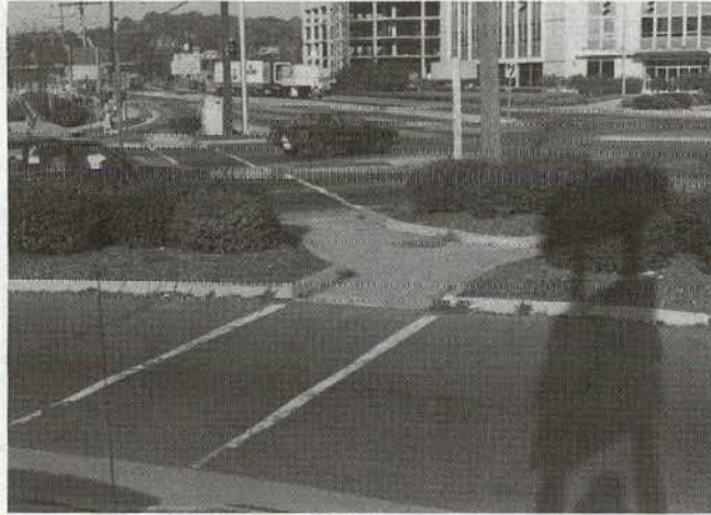
Turning island is unusually well-designed for peds, and encourages proper crossing behavior. Paved crosswalks will be added at this intersection.
