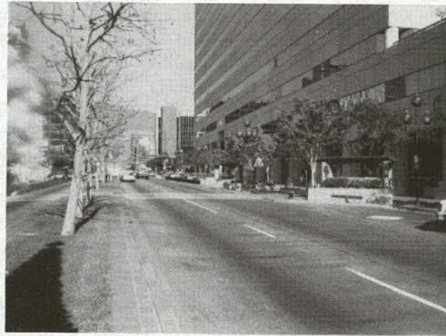
Brand Boulevard, a wide arterial, has been redesigned to better accommodate the pedestrian. A median equipped with curb cuts, landscaping and brick pathways has been provided.
