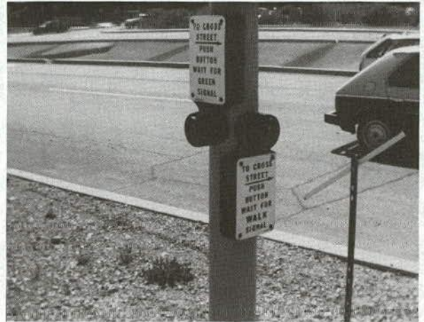
Most signalized intersections have pedestrian actuation. Note arrows indicating direction corresponding to each button. This is often neglected in some cities.
