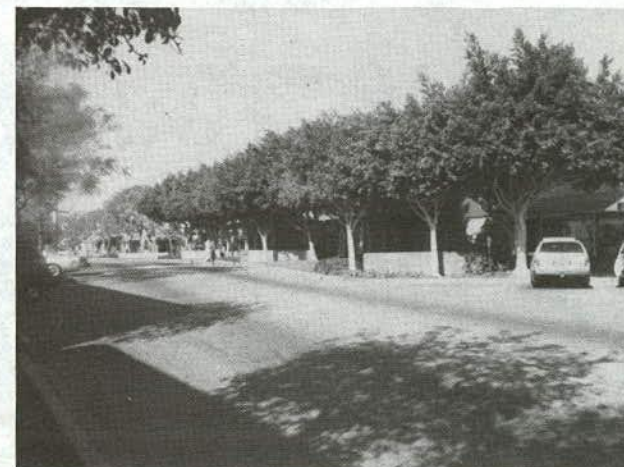
Landscaping and brick walls serve as vehicular barriers.
