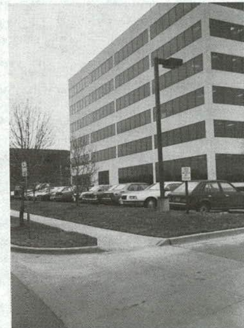
Buildings can be accessed from the sidewalk only through the parking lot.
