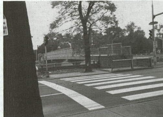
This design provides a landing and barrier to remind pedestrians to stop, look, and think before they cross.
