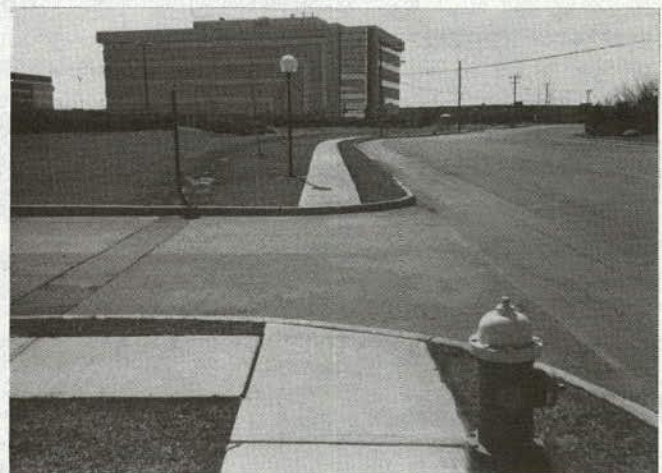
Break in sidewalk for driveway. Note absence of ramped curbs.
