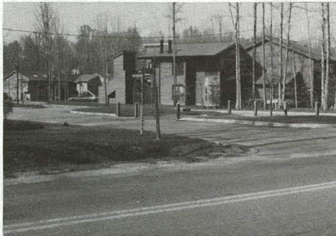
This entrance treatment to one of the neighborhoods slows vehicles and provides a distinctive appearance.
