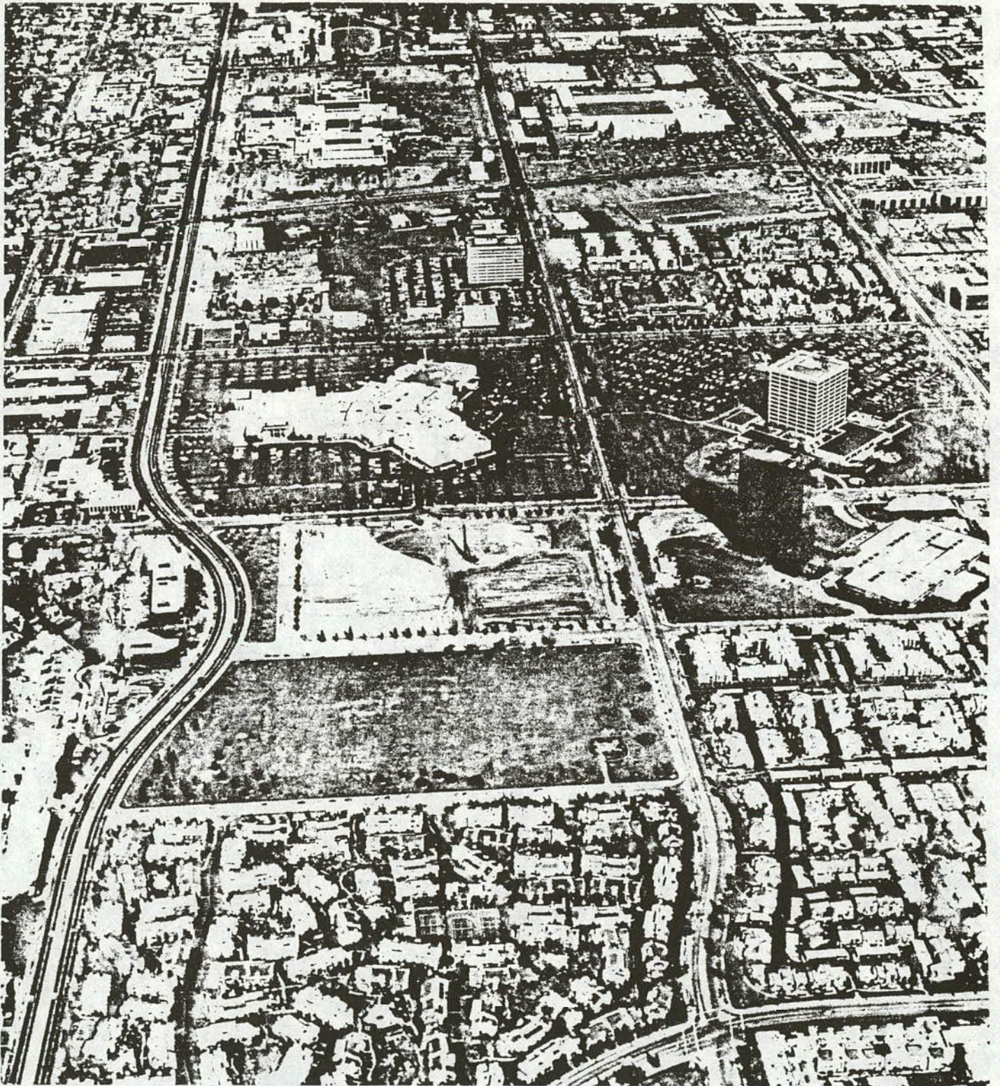
Aerial View of Warner Center
