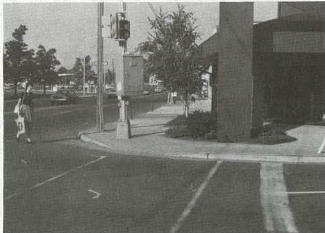
Wilson Boulevard is difficult to cross, except at signals, and could be provided with refuge islands or a narrow median at selected points. Spot landscaping has reduced starkness of wide sidewalk. Controller cabinet impinges on ped path and might have been better placed on opposite side of pole.
