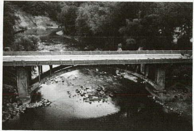
Figure 8. Spandrel arch bridge. (Photo Courtesy of Burgess & Niple, Limited)
