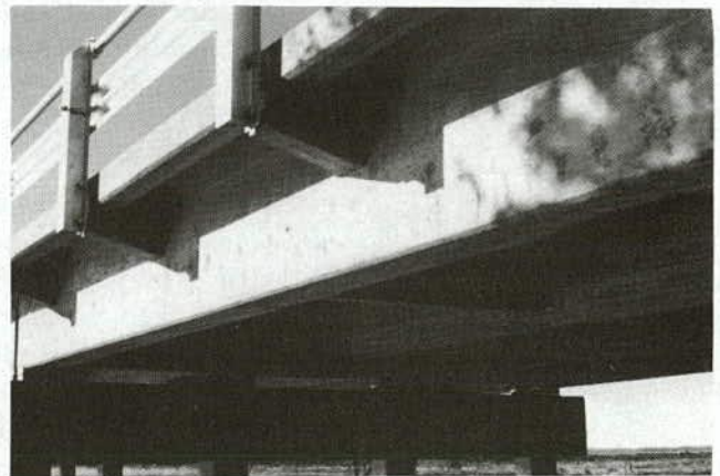
Figure 2. Typical T-beam bridge.
