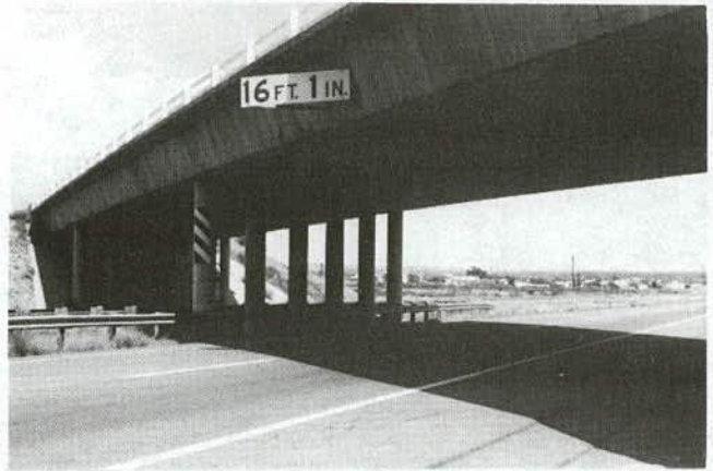
Figure 4. Large concrete box bridge.
