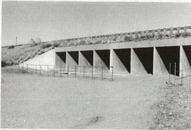
Figure 7. Concrete box culvert.
