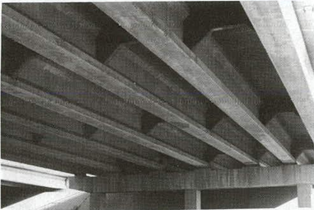
Figure 3. Prestressed girder bridge.
