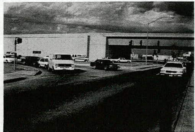
Figure 38. Signalized, dual lane, off ramp right-turn movement.
