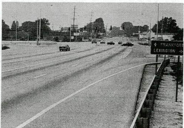
Figure 18. Cross-road right-turn lane.
