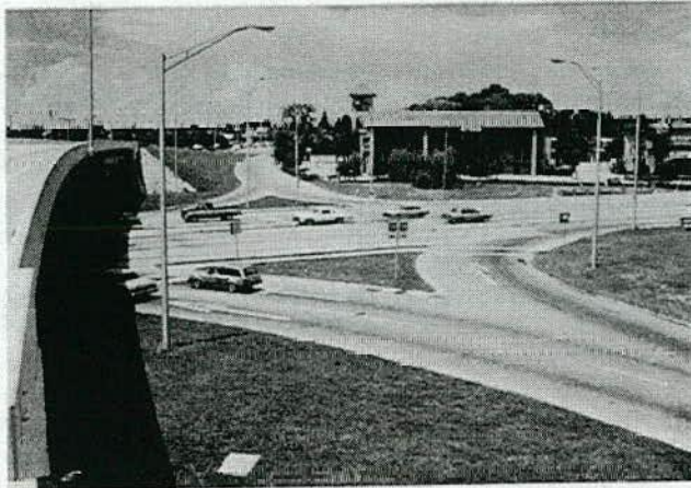
Figure 19. Off-ramp right-turn lane.
