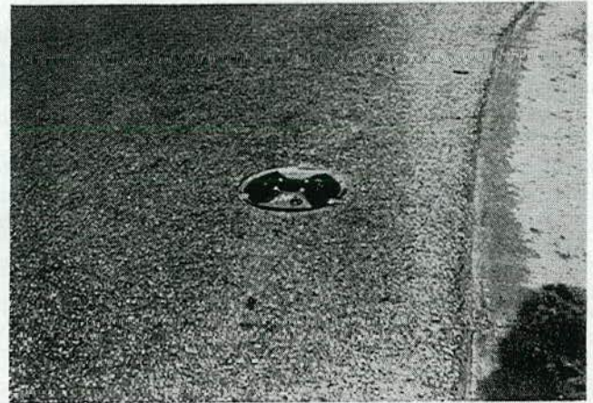
Figure 59. FAA standard runway marker lights used for lane lights.
