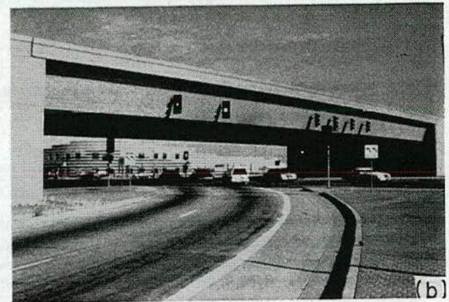
Figure 68. Sight distance through the grade separation structure: (a) structure with open-end spans; (b) structure with closed abutments.
