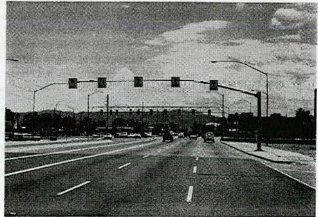
Figure 45. Traffic control device applications at underpass SPUI.
