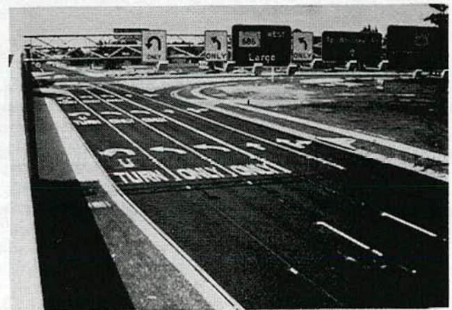
Figure 51. Example of frontage road guide signing application.
