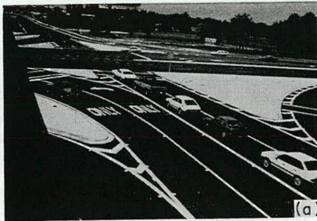
Figure 47. Pavement marking applications: (a) with center island; (b) without center island.
