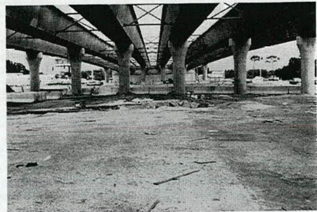
Figure 90. Steel trapezoidal box girder for SPUI bridge under construction.
