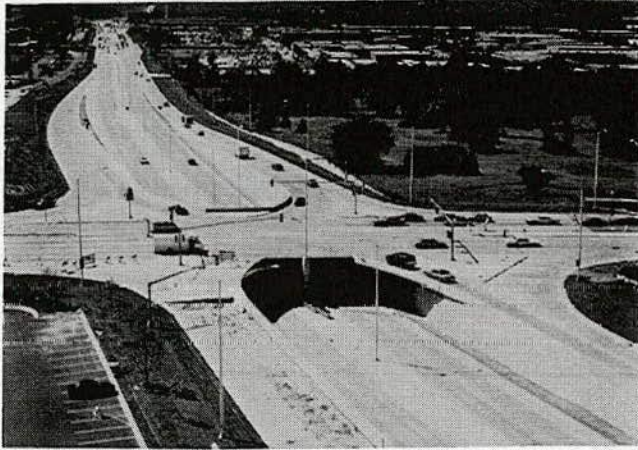
Figure 3. Underpass single-point urban interchange.
