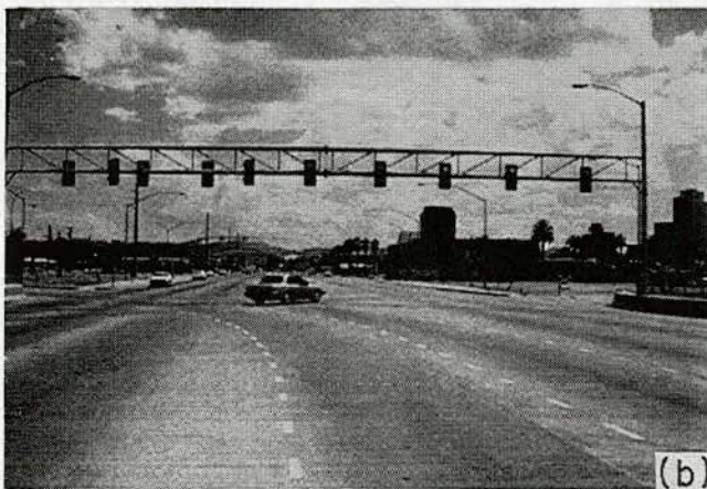
Figure 57. Examples of traffic signal placement for underpass designs: (a) simple span wire design; (b) small steel truss design.
