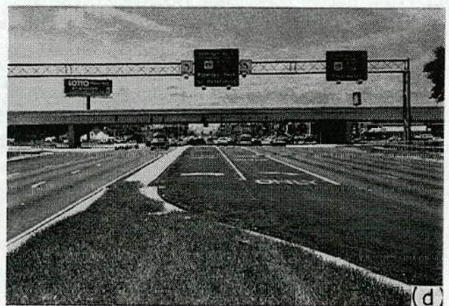
Figure 49. Examples of guide signing applications on cross street: (a) in developing rural area; (b) on suburban arterial; (c) on major urban arterial; (d) high-speed major urban arterial.
