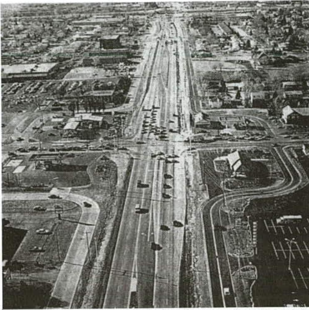
Figure 8-7. Divided arterial streets with 2-way frontage road.
