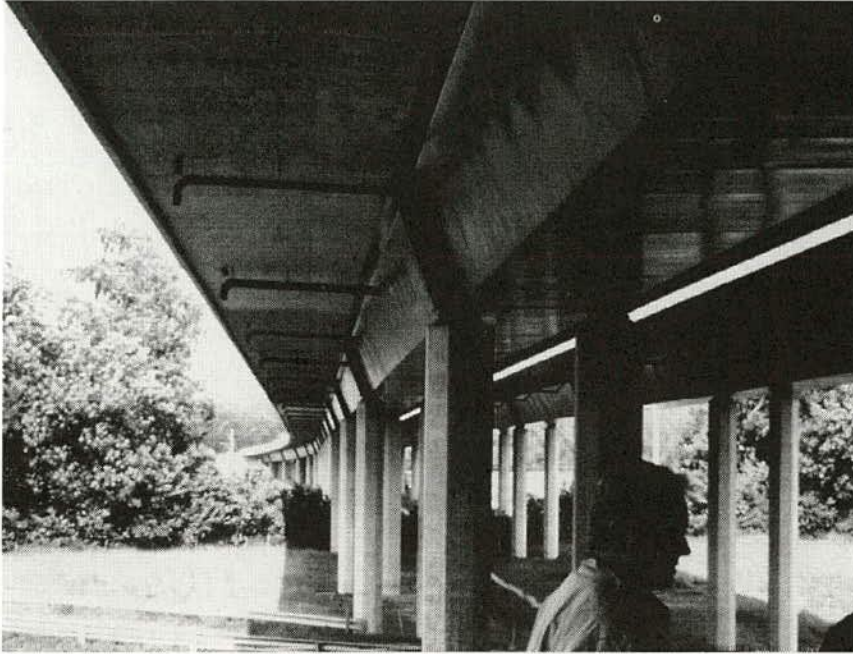
Figure 10. The Viaduct of Bois de Rosset.
