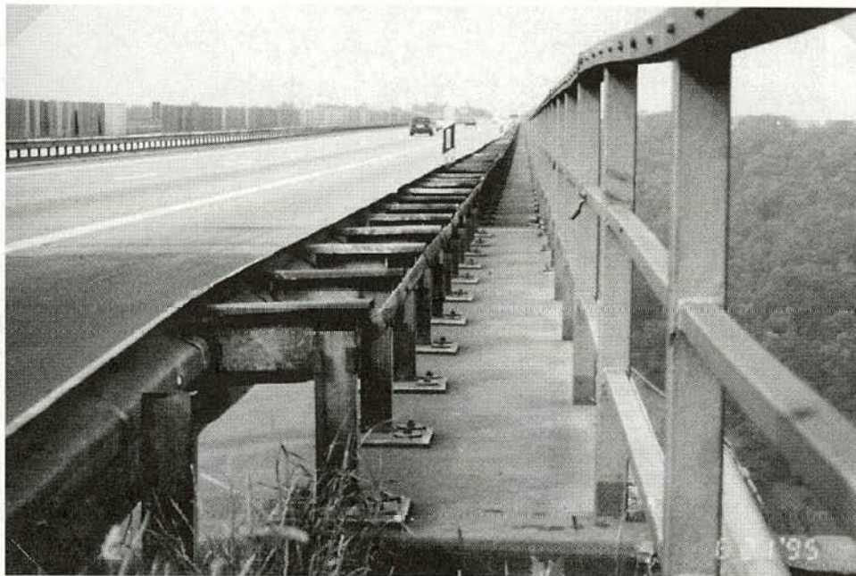
Figure 22. Redundant bridge railings on the Mosel Valley Bridge in Germany.
