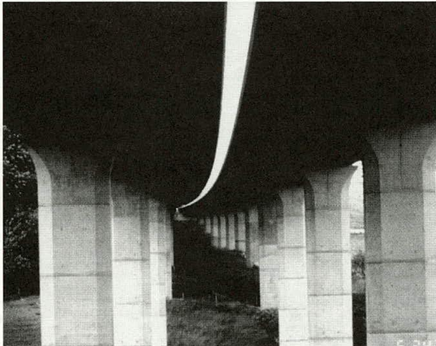
Figure 9. The Viaduct of Löwenberg.
