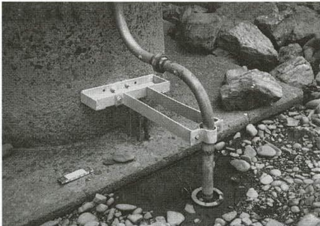
Figure 45. Sliding collar installed upstream of bridge pier at State Route 30/145 over Schoharie Creek at Middleburg, NY.
