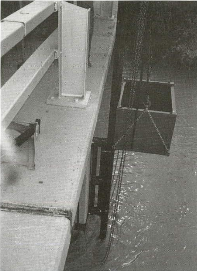
Figure 52. Sonar pipe attached to mounting bracket (Site NM2).
