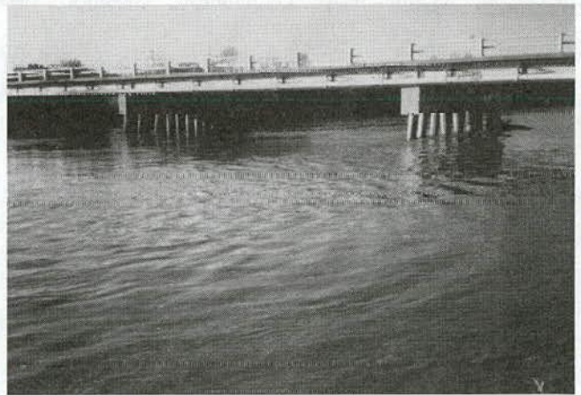
Figure B-11. San Antonio bridge piers (NM2).
