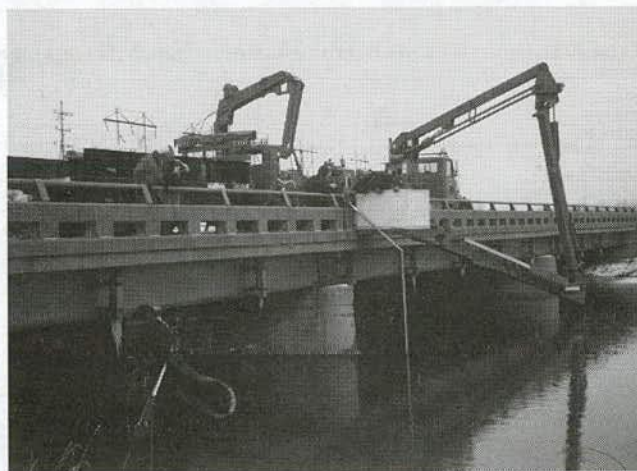
Figure 33. Installation of offset for sliding collar device (Site M11).
