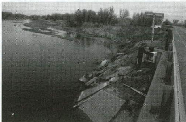
Figure 26. Sonic instrument (black rod), sliding collar (cable), and data box at Kersey bridge (Site CO2).
