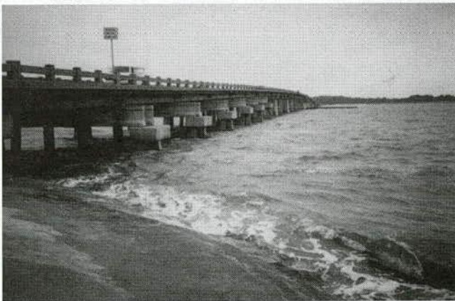
Figure B-18. South abutment, Nassau Sound bridge looking to the north.
