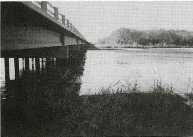
Figure B-9. Bernardo bridge piers (NM1).
