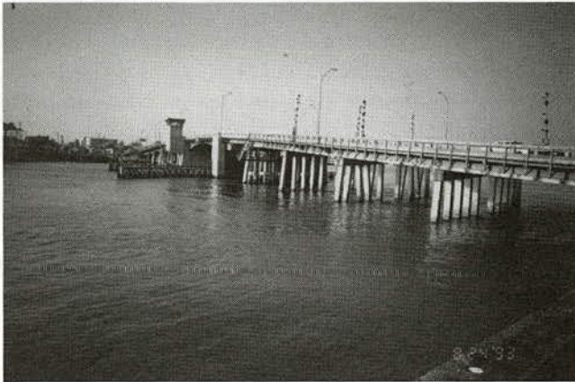
Figure B-14. Johns Pass bridge near St. Petersburg, Florida (Site FL1).
