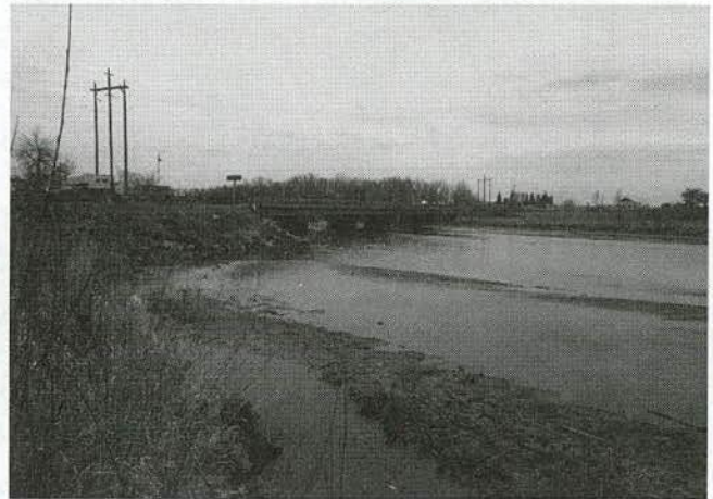
Figure B-6. Overview of Kersey bridge (Site CO2)-looking downstream.
