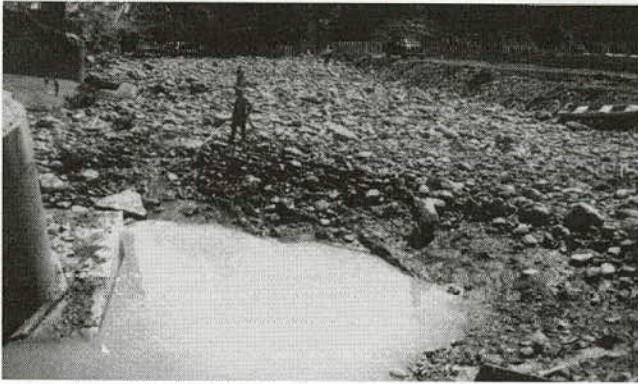
Figure 75. Configuration of the local scour hole at Pier 2, Schoharie Creek, NY, 1987.
