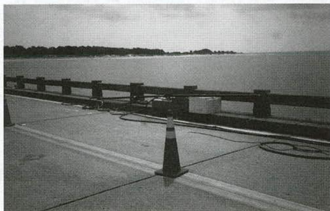
Figure 27. Overview of Nassau Sound automated sliding collar with driving extension (Site FL2).
