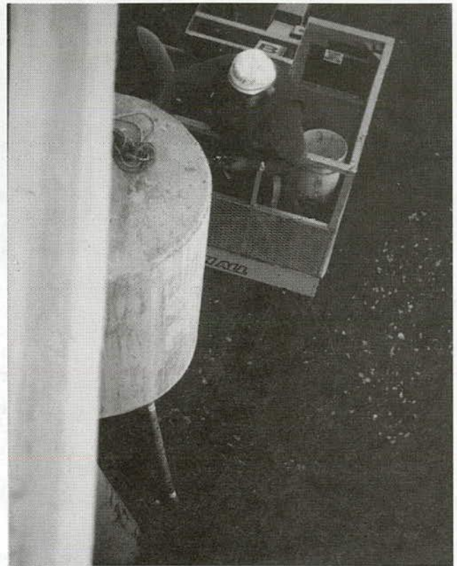
Figure 40. Installation of sliding collar device at Minnesota bridge no. 23015 (Site MN2).
