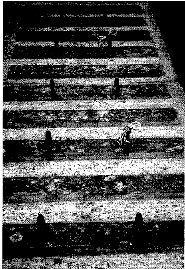
Figure 4. Shear keys on concrete I-girder.
