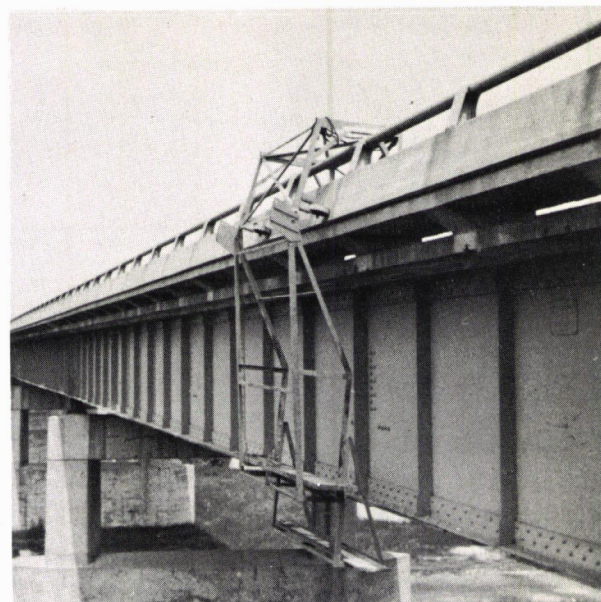
Figure 6. Rolling bridge-painting scaffold developed by maintenance personnel (Test Section 59, Ohio Turnpike).
