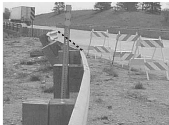
Figure 51. Measuring Rail-Height Post Deflection
