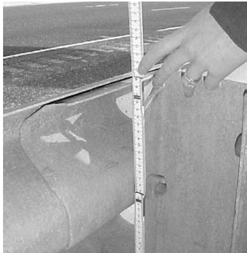
Figure 28. Rail Height (close-up)
