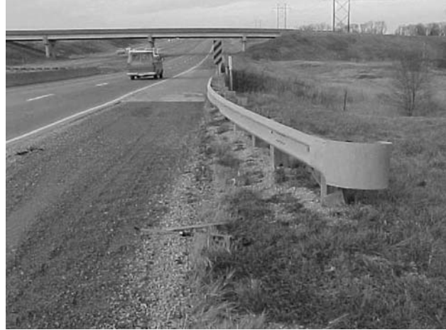
Figure 73. Example Iowa Wood-post BCT
