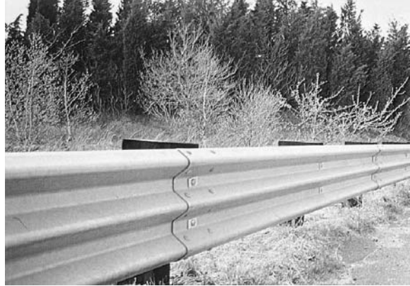
Figure 40. Three Beam with Wood Posts
