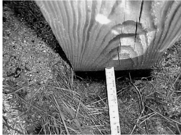
Figure 48. Measuring Groundline Post Deflection
