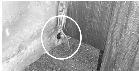
Figure 55. Splice Failure
