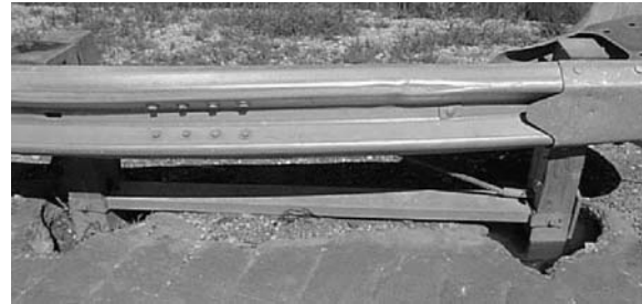
Figure 47. Groundline Strut
