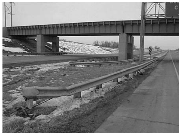
Figure 20. Downstream View of Scene
