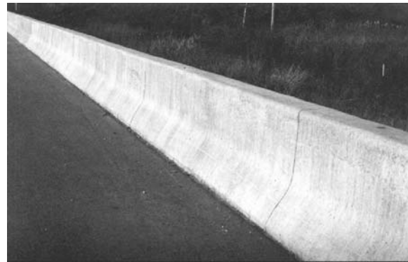
Figure 65. Concrete Safety Shape Barrier
