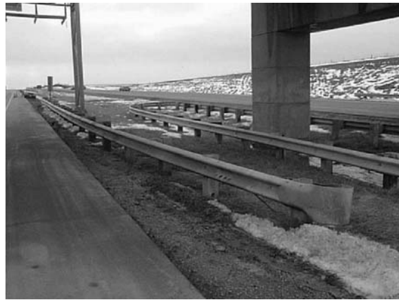
Figure 19. Upstream View of Scene
