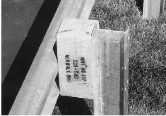
Figure 39. W-Beam, Steel Post and Wood Blockout
