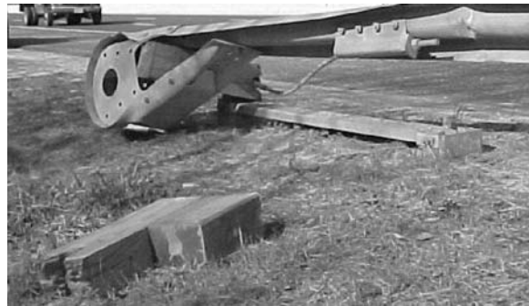
Figure 52. Broken Wood Posts
