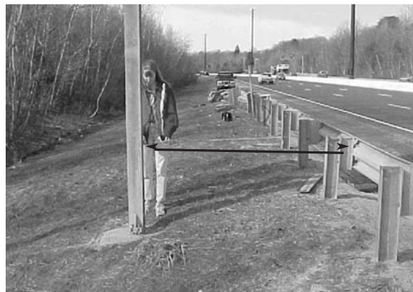
Figure 31. Offset to Nearest Hazard.
