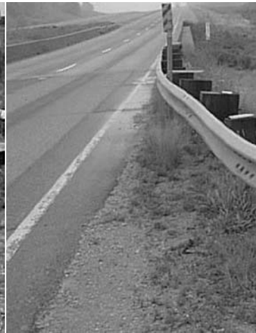
Figure 37c. Partially Paved Shoulder
