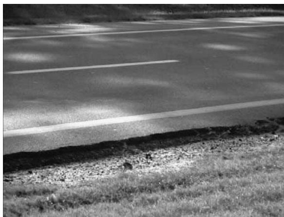
EXHIBIT V-15 Example of an Edgedrop
