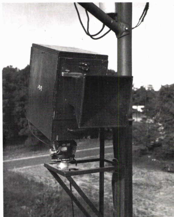
CLOSEUP VIEW OF COMPLETED INSTALLATION
