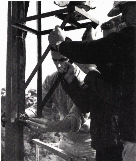
SECURING POLE BRACKET TO LIGHTING STANDARD
