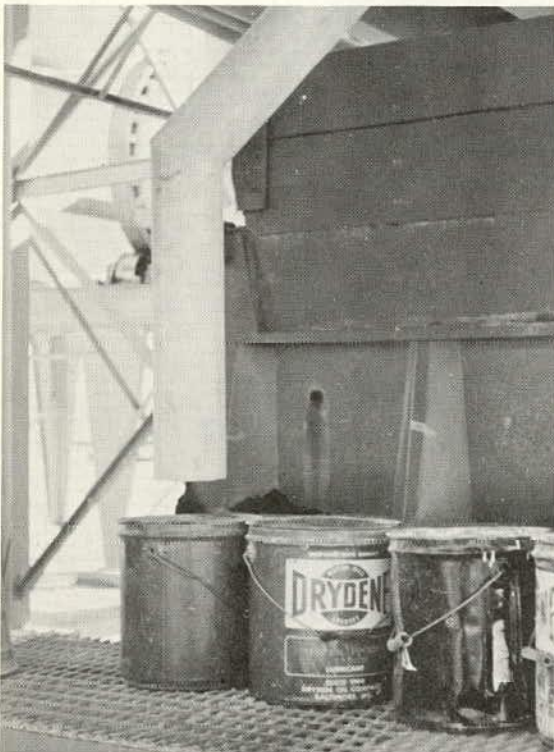
Figure 18. Sampling chute and containers, Plant No. 3.
