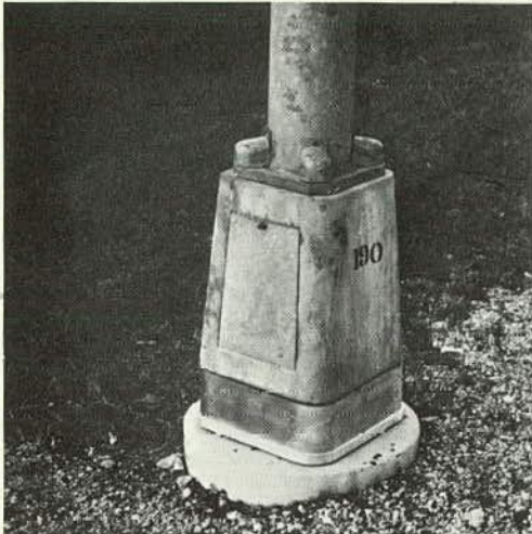
Figure 8. Cast aluminum insert with steel T-base.
