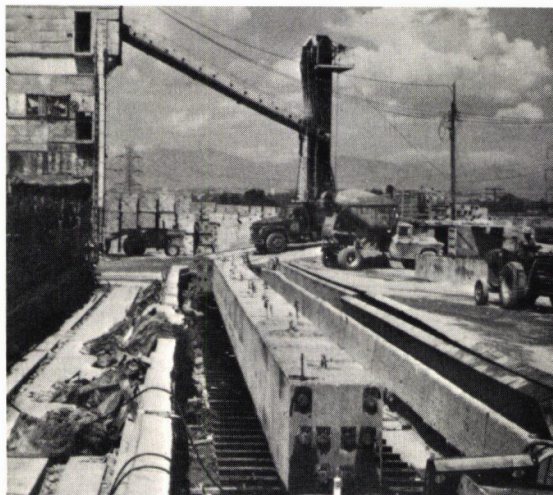
Figure G-14. Girder after removal of forms.
