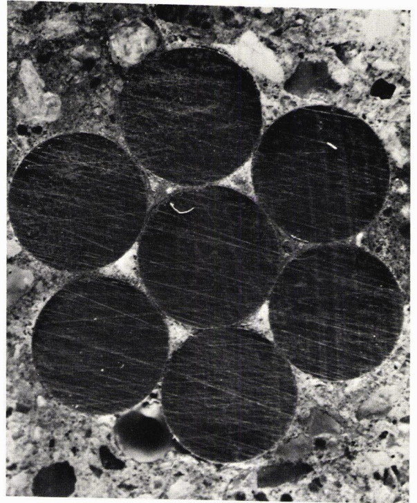
Figure H-1. Section of 0.5-in. strand in pretensioned girder fragment after 1½ years on bank of South Platte River, Ft. Morgan, Colo. Note cement paste in strand interstices.
