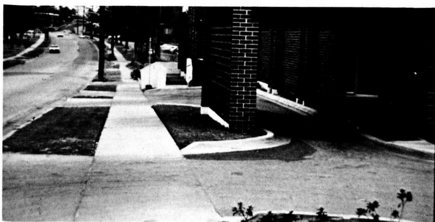
Figure 22. Drive-in service window and driveway with restrictive turning radii and limited storage for queued vehicles.
