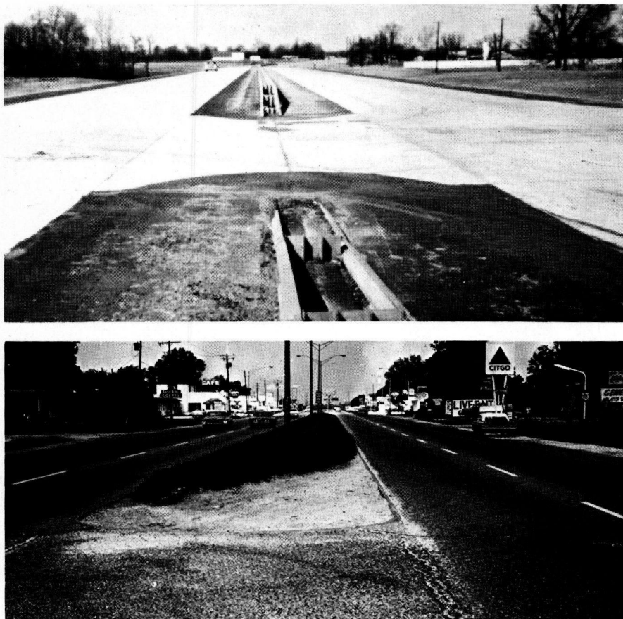
Figure 9. Circular end treatment of median openings. On this newly opened facility near Indianapolis (upper), the paths of vehicles turning left from the right-hand roadway to a local gravel road to the left of the photograph follow a natural spiral using a portion of the median outside the portland-cement-paved median crossing. In this instance the median has an asphalt surface so that erosion of the median surface will not be a problem (unless, of course, the repeated wheel loads cause breakup of the asphalt surface). Median crossings on Airline Highway (lower) have circular end treatment at median openings. Left-turning vehicles entering the northbound roadway follow a natural path across the grassed median; although the gravel surface is rough, it is the preferred path.
