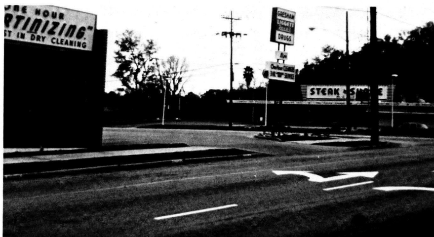
Figure 21. Inadequate corner clearance for exit driveway.
