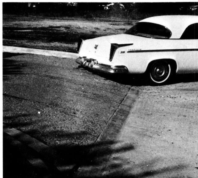
Figure F-13. Adverse driveway profile. The grade change is so severe that the vehicle must cross the curb line at an angle to avoid dragging the rear bumper.
