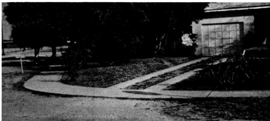
Figure F-10. Example of a poor residential driveway. This driveway is too narrow to provide a convenient walkway for persons entering or leaving the vehicle. Because the driveway opens into the intersection between a local and a collector street, to exit from the driveway it is necessary to back into the street. The hazard of this maneuver is compounded by visibility restrictions imposed by the shrubbery.
