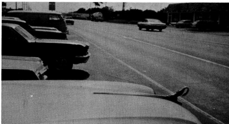
Figure 12. Restricted sight distance due to improper parking at commercial development with open frontage.
