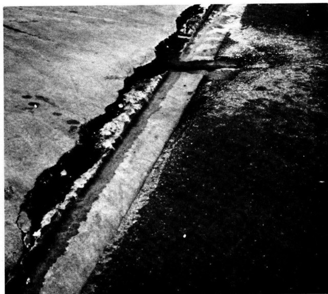
Figure 19. Spalling at driveway due to poor construction practices in making the curb cut.
