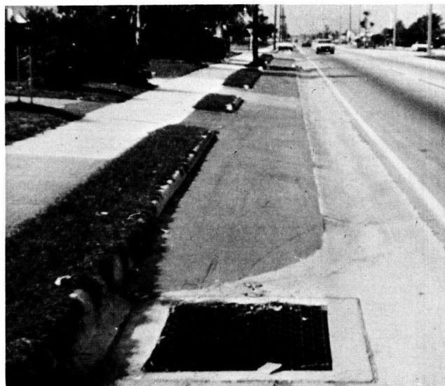
Figure F-17. Discontinuities of driveway profile across gutter along arterial roadway.
