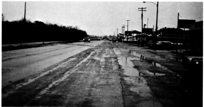
Figure F-19. Unsatisfactory driveway surfaces. Unpaved commercial driveway along an arterial (upper). Poor maintenance of commercial driveways (lower).
