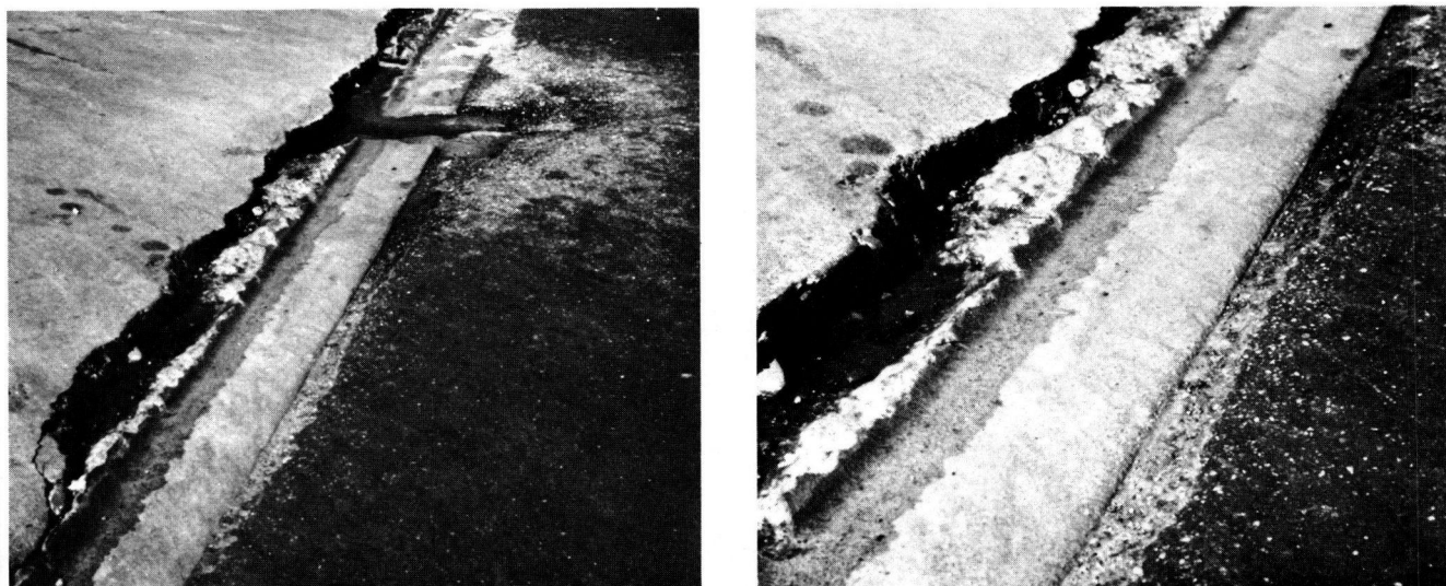
Figure F-20. Poorly constructed curb cuts. Such curb cuts may lead to the formation of large spall areas which are unsightly and a maintenance problem. To avoid this problem, the entire curb and gutter section should be removed when the curb cut is made.
