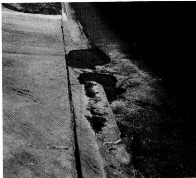
Figure 18. Potholes along curb line of poorly maintained driveway.
