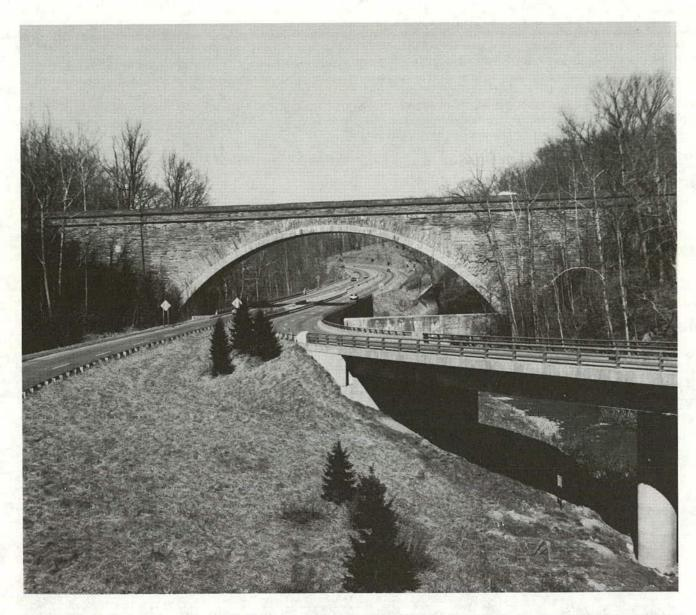
FIGURE 9 Cabin John Aqueduct (1853-1863), Glen Echo, Maryland. The deteriorated stone parapets and masonry shadow course were replaced by pigmented precast concrete. (Photo by Eric DeLony, HAER.)
