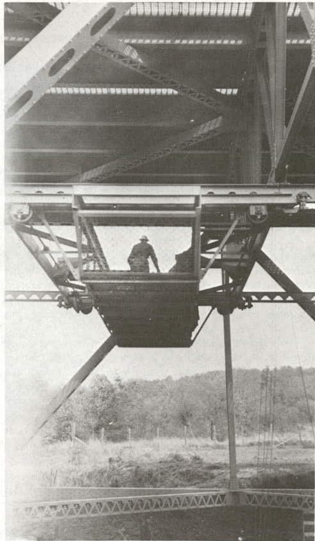
FIGURE 1 Tacoma Narrows Bridge—through traveler.
