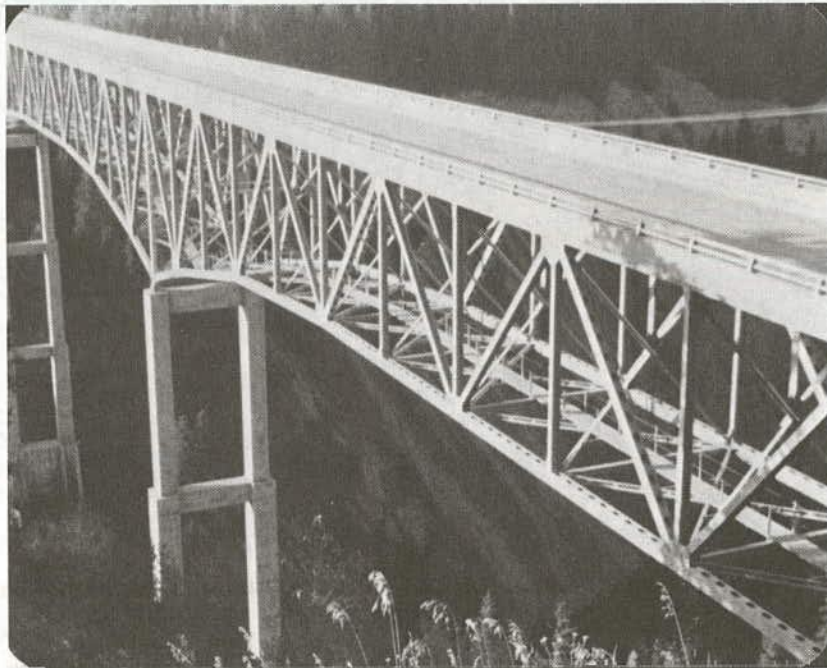
FIGURE 3 Idaho Bridge—timber walkway.
