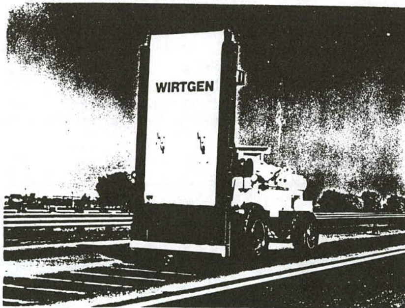
FIGURE 5 A guillotine concrete-shattering machine.
