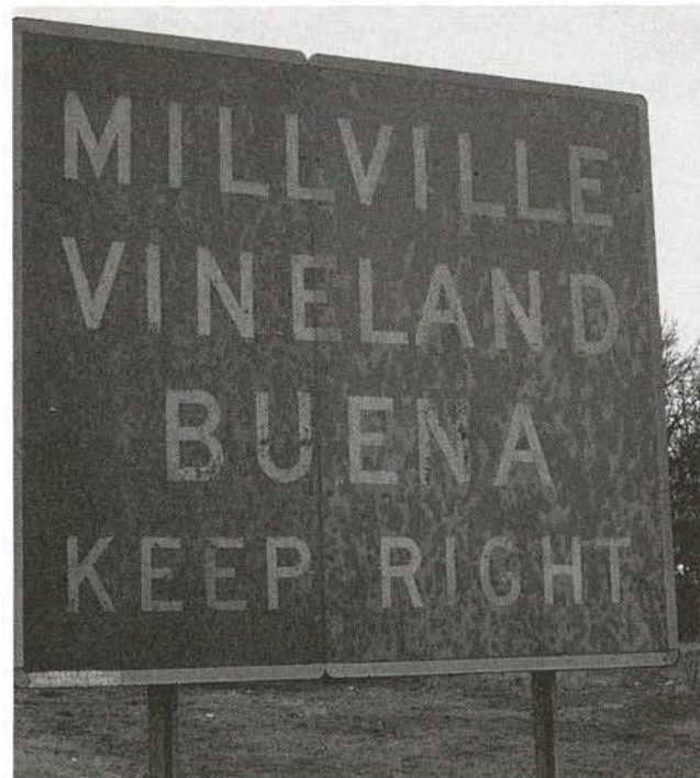
FIGURE 1 Examples of deteriorated guide signs.
