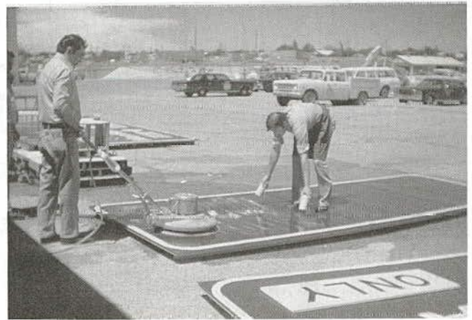
FIGURE 21 Sign blank scrubbed with floor polisher and powdered chlorinated cleaner.
