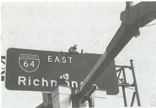
FIGURE 17 Illustration of overlay method of sign refurbishing.
