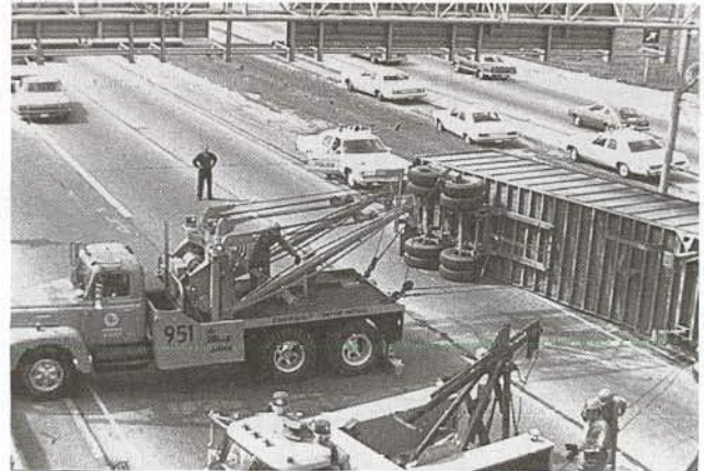
FIGURE 6 Incident removal using heavy-duty tow trucks.
