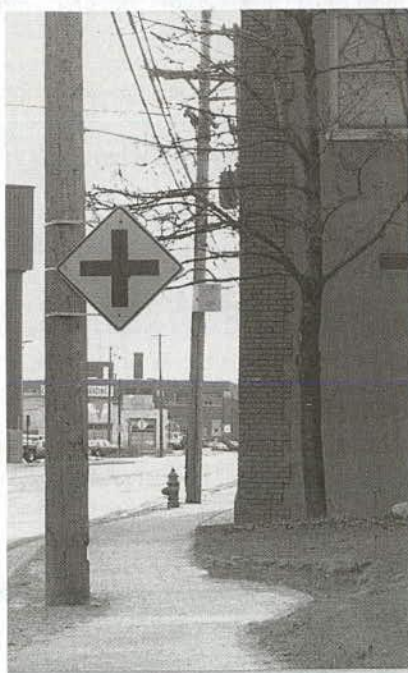
FIGURE 6 Sign mounted on a utility pole.
