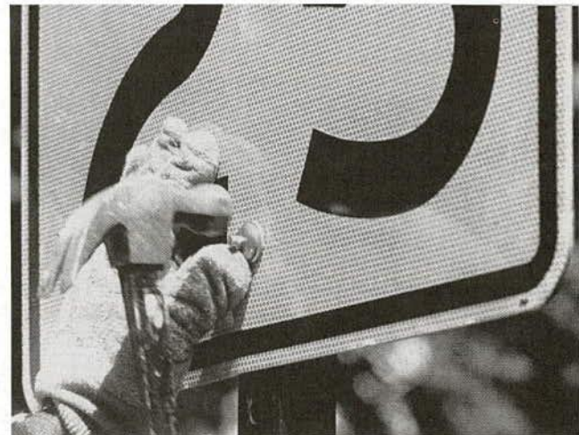
FIGURE 48 Vandal-resistant fasteners.
