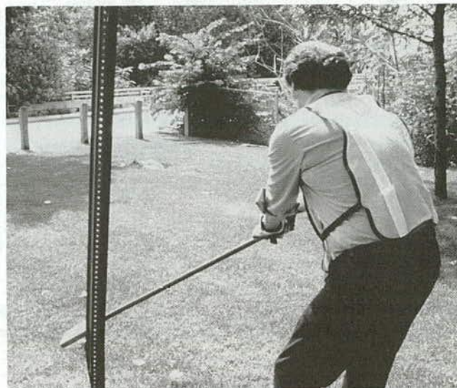
FIGURE 10 Signpost being straightened.
