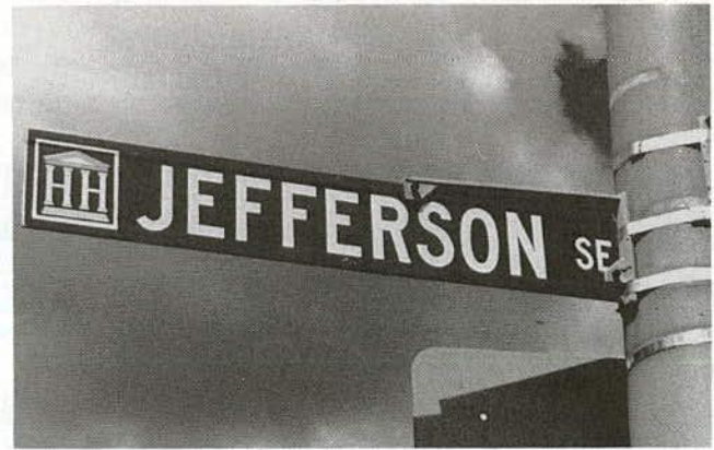
FIGURE 47 Sign mounted on utility pole with SIGNFIX.
