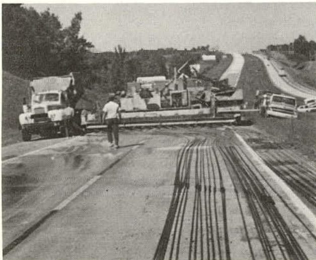
Figure 7. CRC overlay construction.
