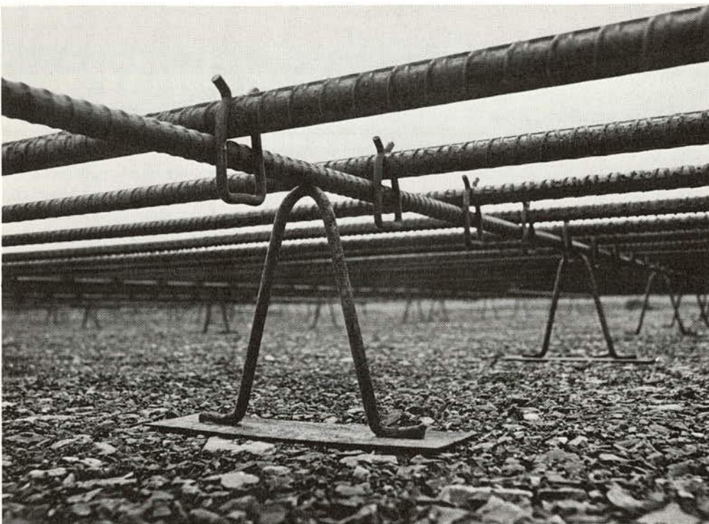
Figure 9. Continuous high chair with welded clips.
