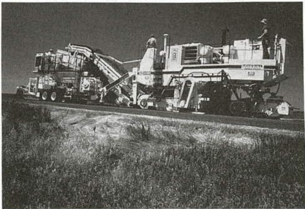
FIGURE 17 Cold-milling machine with portable crusher (CMI).
