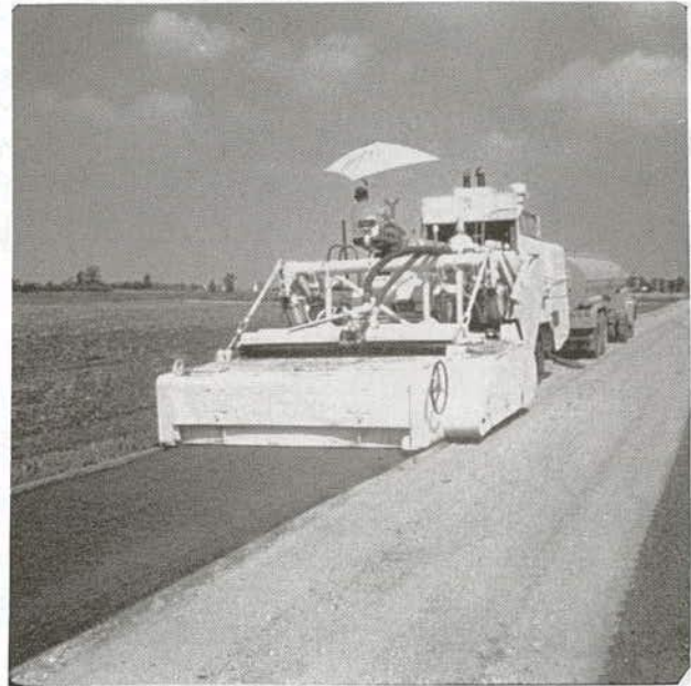
FIGURE 26 Multiple transverse-shaft rotary mixer.
