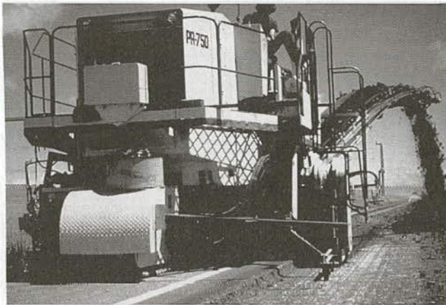
FIGURE 10 Cold-milling machine for pavement removal and sizing.
