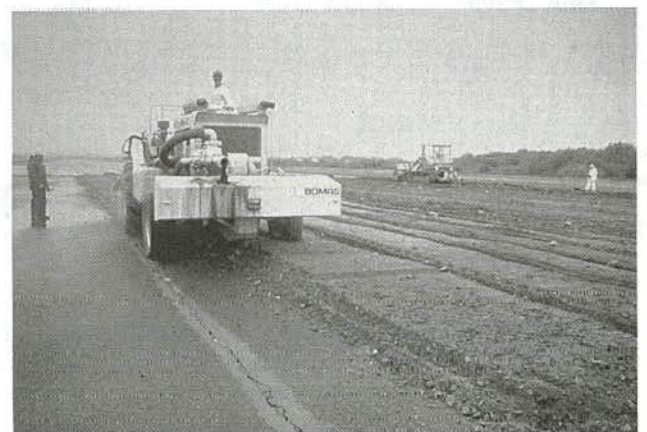
FIGURE 7 Single-shaft rotary mixer for size reduction.
