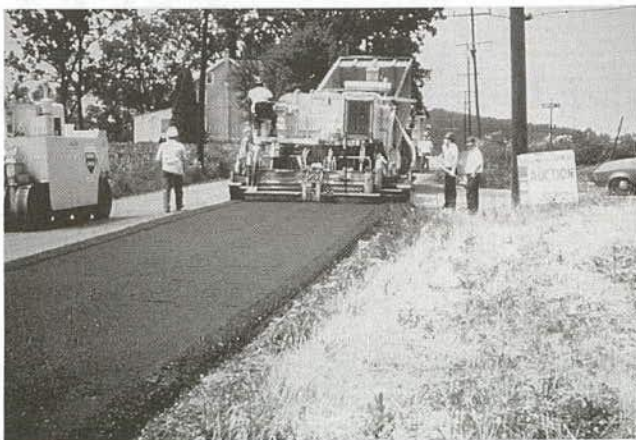
FIGURE 29 Laydown of cold-recycled base using Midland Motopaver.
