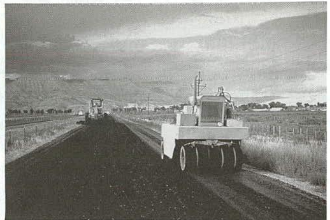
FIGURE 30 Pneumatic-tired roller for compaction.
