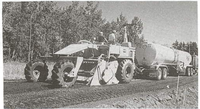
FIGURE 12 Soil stabilization mixing equipment for adding stabilizer.
