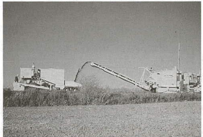
FIGURE 13 Traveling mixer adding stabilizer to recycled asphalt pavement from cold-milling machine.
