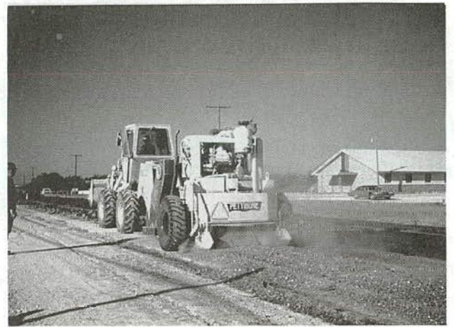
FIGURE 6 Traveling hammermill.
