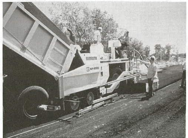
FIGURE 31 Hopper type paver for laydown of surface course over cold-recycled base.
