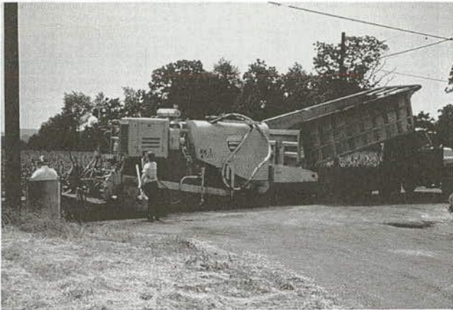
FIGURE 28 Hopper of mixer-paver receiving cold-recycled mix.
