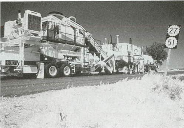
FIGURE 20 Portable crusher attached to cold-milling machine.
