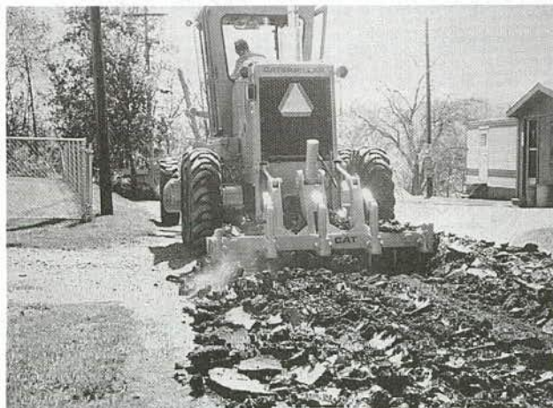
FIGURE 5 Motor grader with cutter-crusher-compactor.
