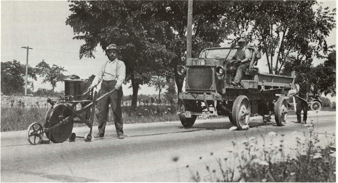
Figure 1. Hand-powered striper. (Wisconsin Dept. of Trans.).
