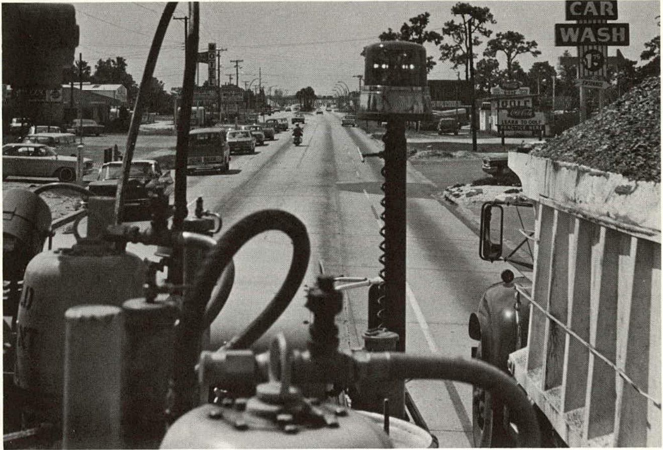
Figure 11. Traffic situation requiring fast-dry heated paint.
