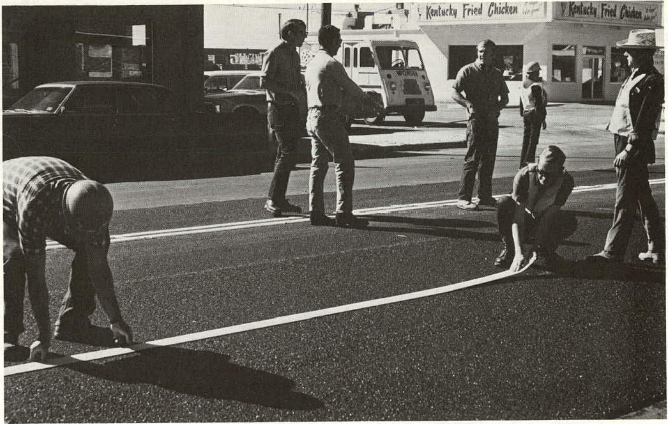
Figure 5. Applying cold thermoplastic stripe.
