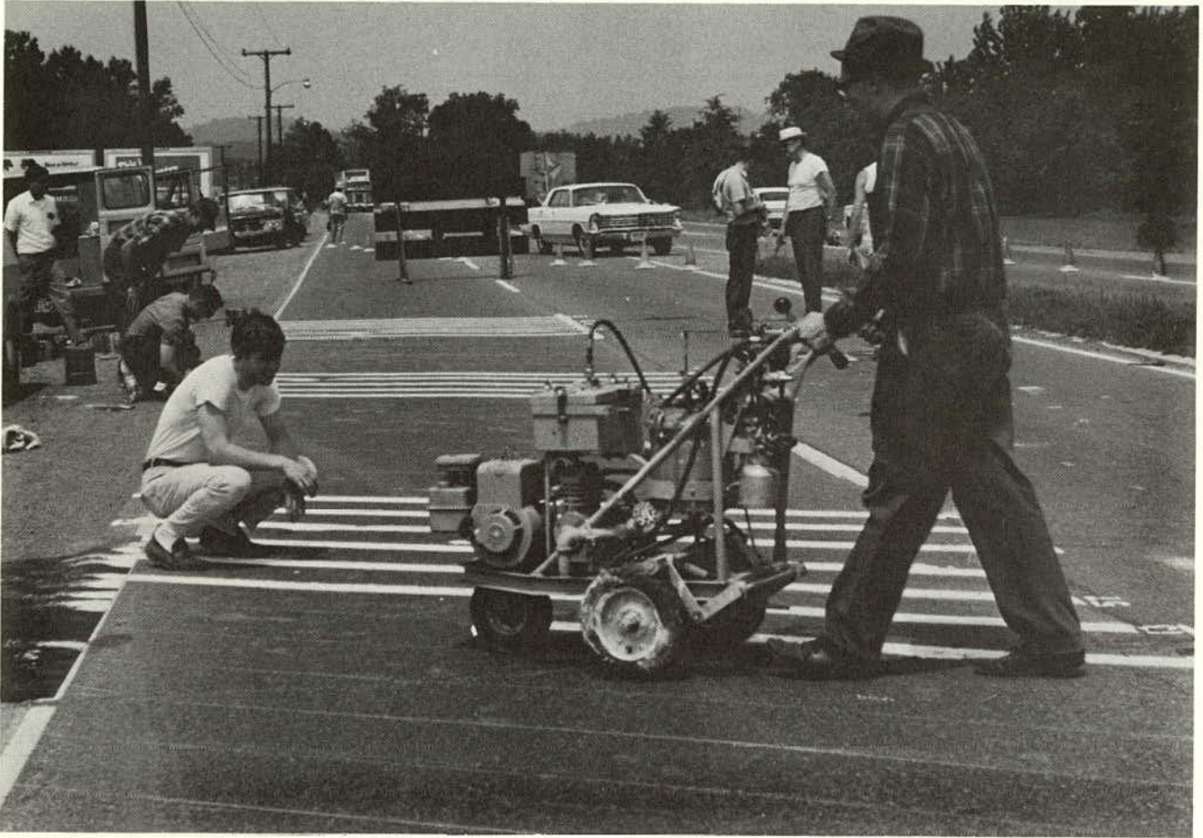
Figure 6. Applying test stripes.
