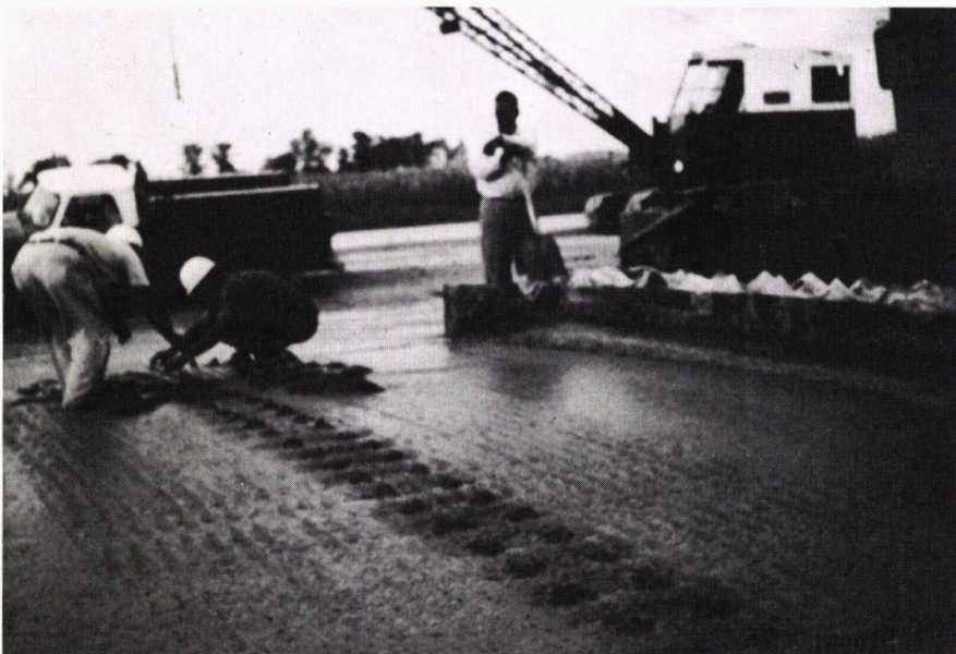
Figure 14. Surface disturbance behind placer.
