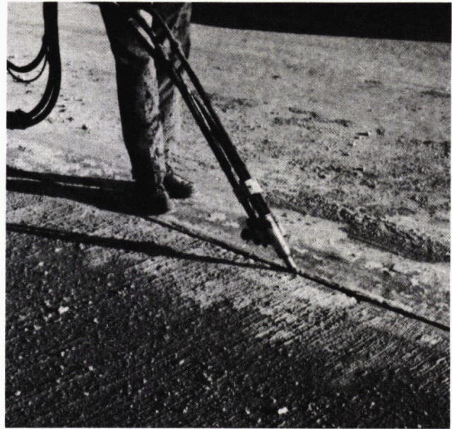
Figure 19. Application of two-component sealant.
