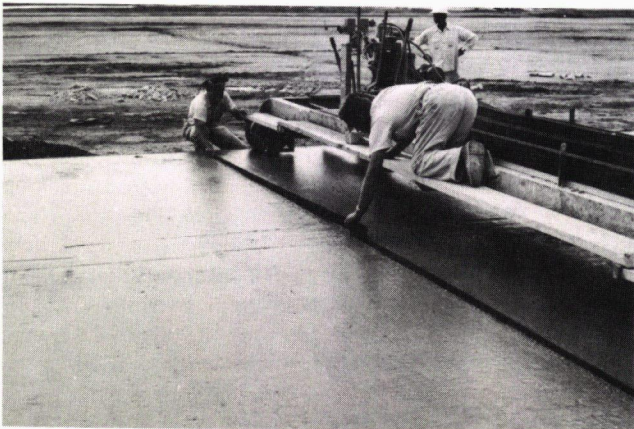
Figure 10. Insertion of strips in transverse joint.
