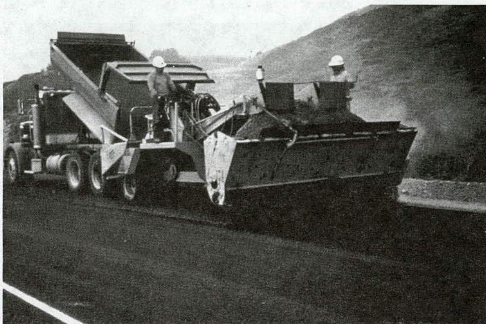
FIGURE 10 Chip distributor.
