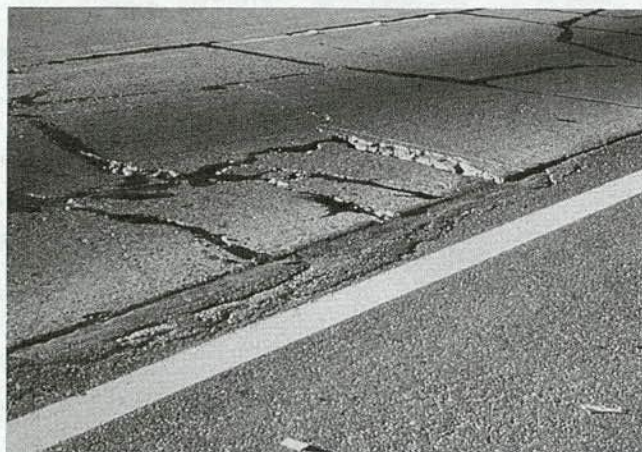
FIGURE 11 Shattered slabs.
