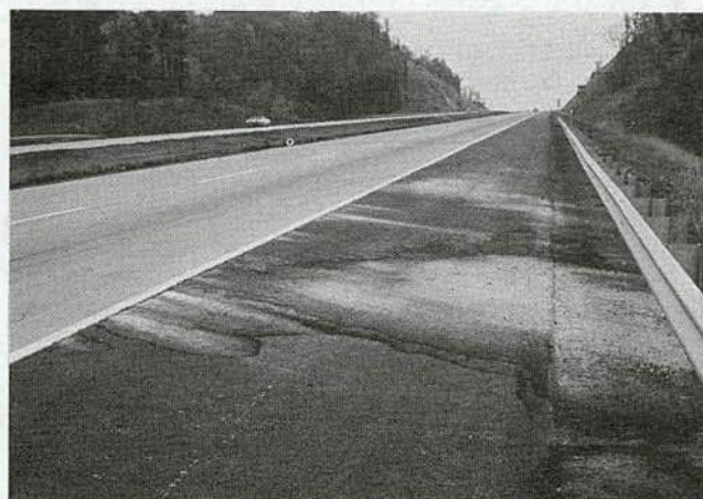
FIGURE 12 Pumping slabs.
