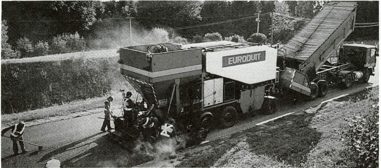
FIGURE 4 NOVACHIP paving equipment.
