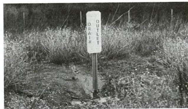
FIGURE 8 Typical outlet headwalls and location marker (7): (a) precast concrete headwall; (b) fabric formed concrete headwall; and (c) delineator post used for marking outlets.
