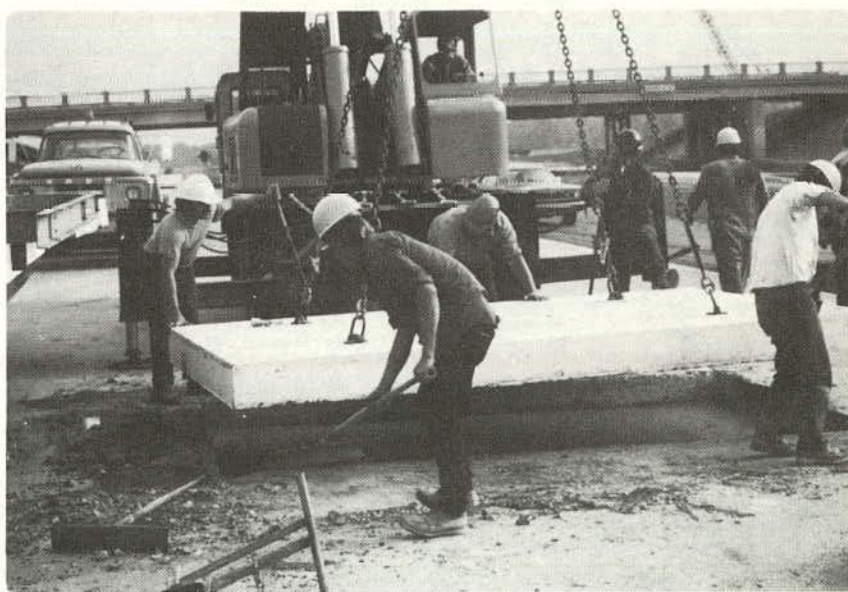
Figure 13. Precast concrete slab being placed at full-depth repair site.
