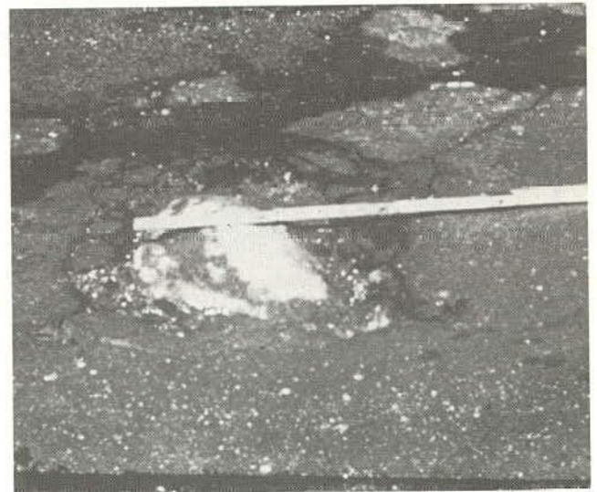
Figure 13. Stone (approx. 9 in.) raised by frost action until it has broken through the pavement surface (28).
