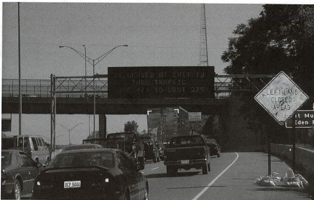
FIGURE 14 The ARTIMIS traffic management system uses several information resources including permanent changeable message signs to inform motorists of alternate routes. (Photo courtesy of TRW, Inc.)
