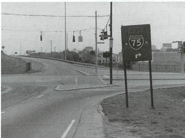
FIGURE 11 Dayton, Ohio, has erected permanent detour signs along six preplanned alternate routes for three sections of I-75 within the city limits. (Photos courtesy of the Dayton Police Department.)
