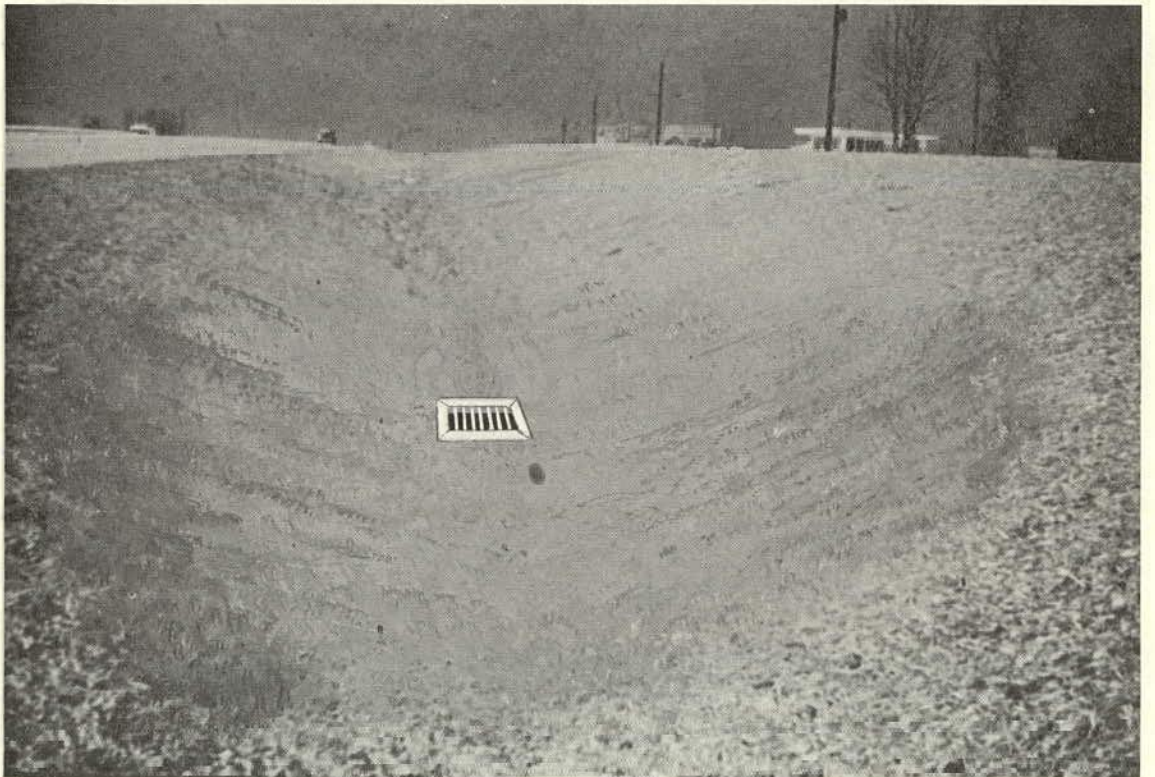
Figure 26. Hazardous drainage practice between two roadways (top). Possible modification with drop inlet and flat slopes (bottom).
