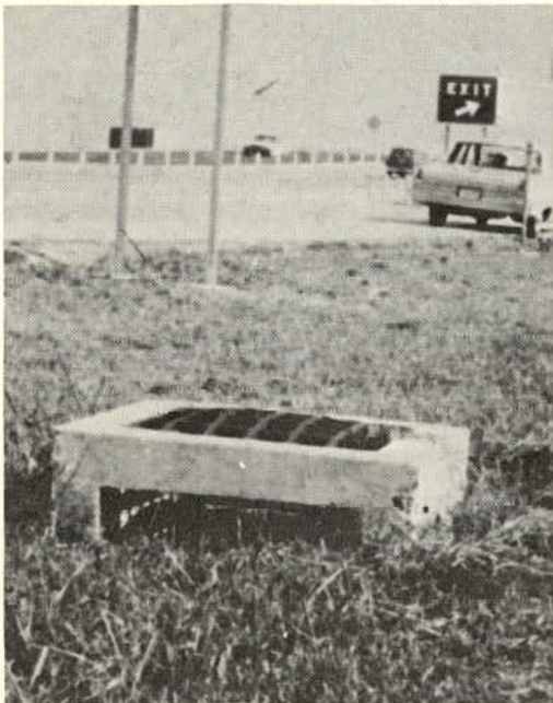
Figure 17. Examples of common median inlets that are potential traffic hazards.
