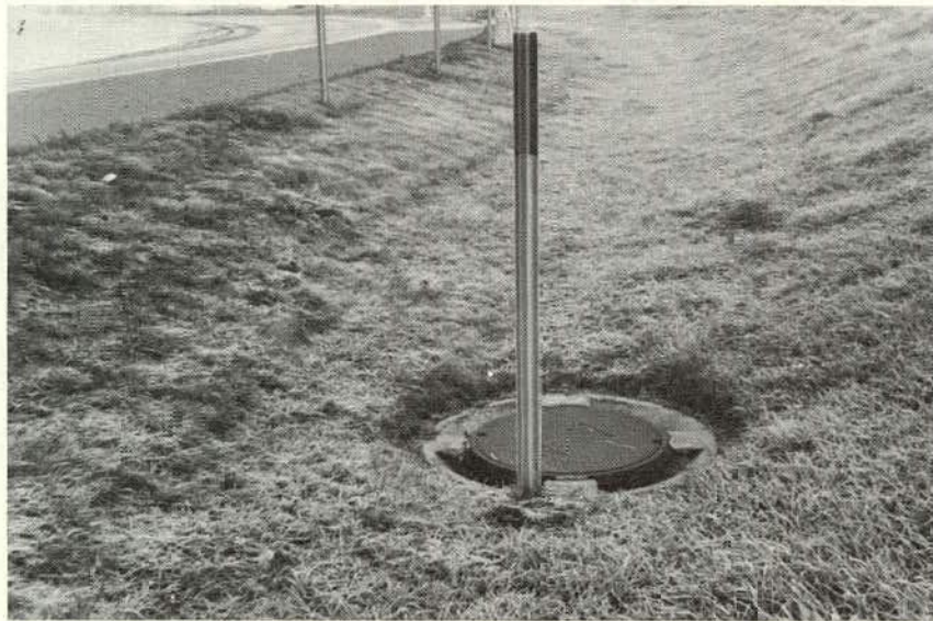
Figure 12. Precast concrete drop inlet with removable cover. Slender post aids location under snow.
