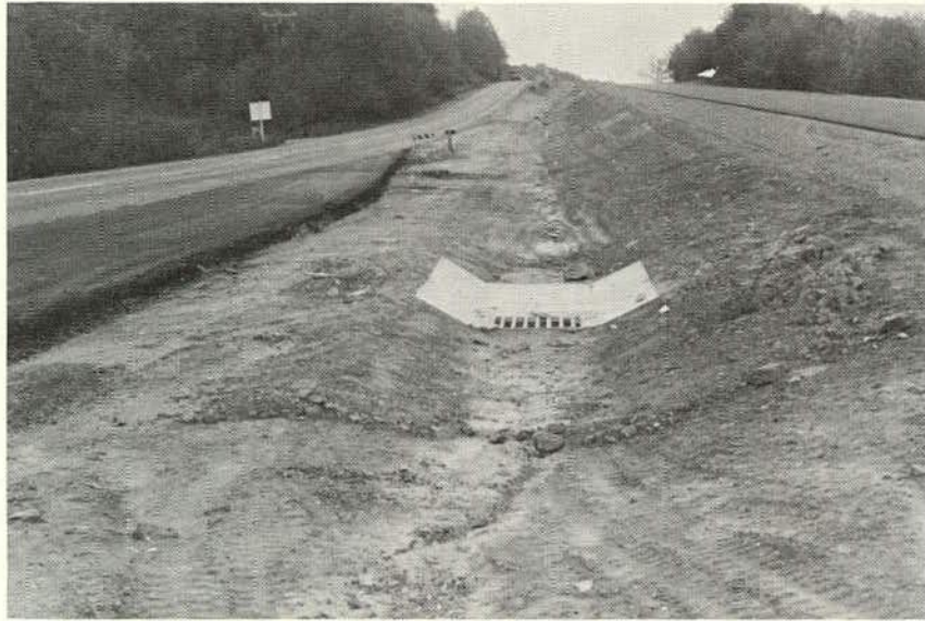
Figure 10. One type of concrete apron to discourage vegetation overgrowth, prevent erosion, and facilitate maintenance.
