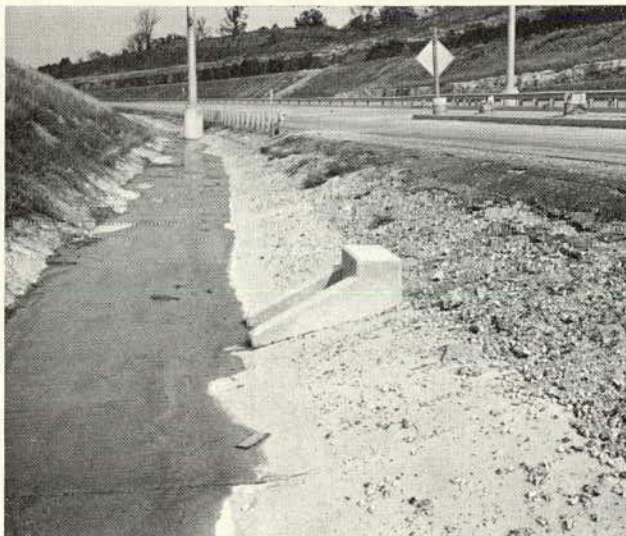
Figure 19. Projecting headwall located within the recovery area.
