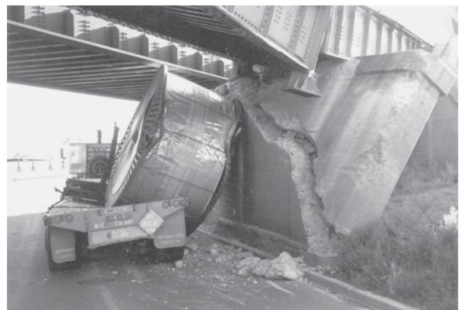
FIGURE 7 Example of vehicle–bridge collision causing collapse owing to nonredundant substructure. (Courtesy: Robert Sweeney.)
