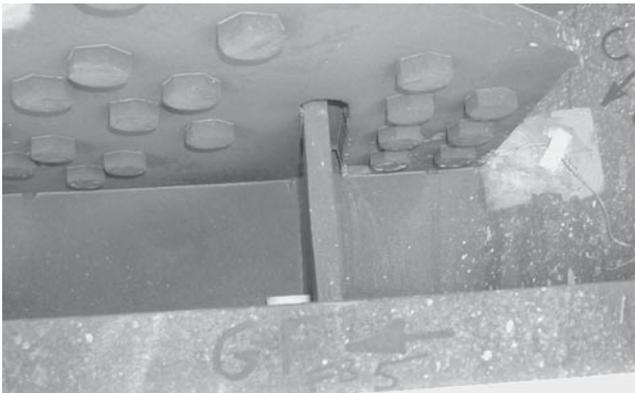
FIGURE A3 Fractured girder of the Hoan Bridge in Milwaukee (top) and view of critical shelf plate detail featuring intersecting welds.
