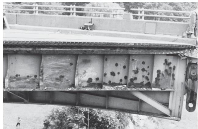
FIGURE 4 Collapse of Mianus River Bridge. (Courtesy: John W. Fisher.)
