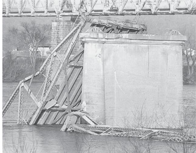
FIGURE 1 Collapse of Point Pleasant Bridge.
