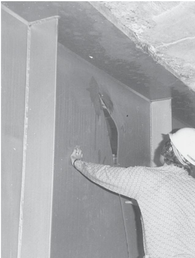
FIGURE A12 Full-girder-depth fatigue crack of Lafayette Street Bridge in St. Paul, Minnesota.
