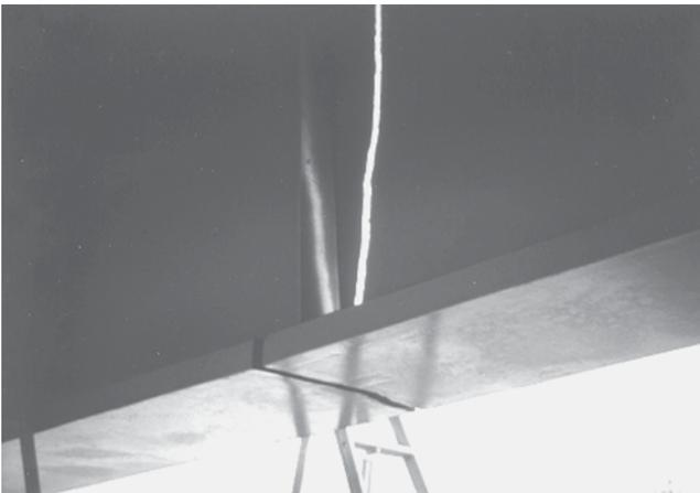
FIGURE 17 View of cracked girder in two-girder span of I-79 Bridge at Neville Island in Pittsburgh as an example of a two-girder bridge that is sufficiently redundant to avoid collapse despite a fracture of the tension flange and the web of one girder.
