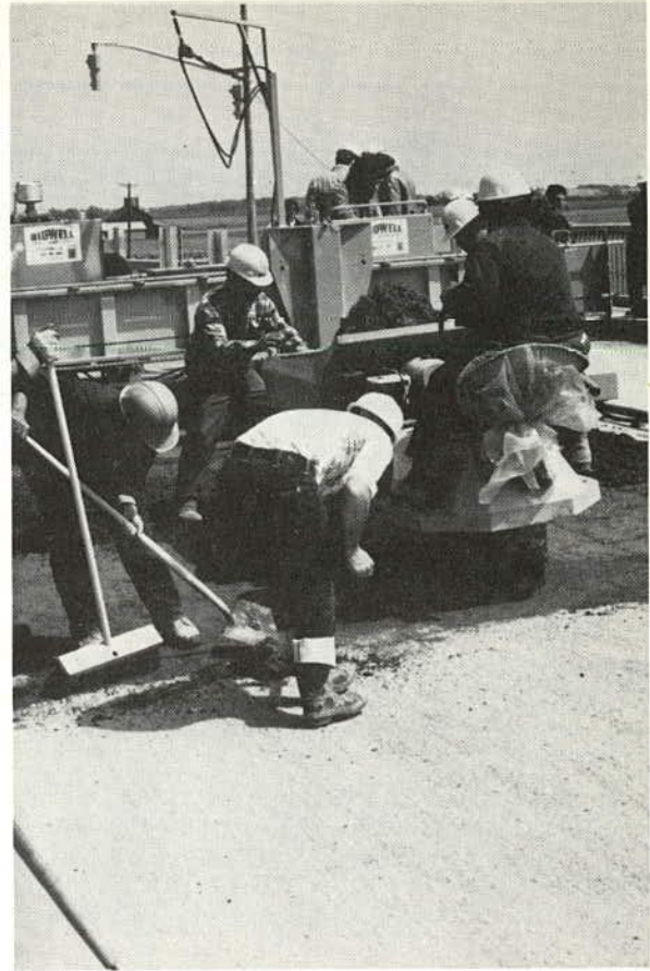
Figure 13. Placement of a low-slump concrete overlay.
