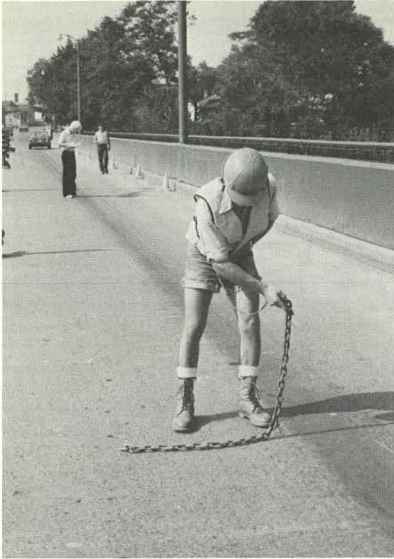
Figure 7. Use of heavy chain for detection of delaminations.
