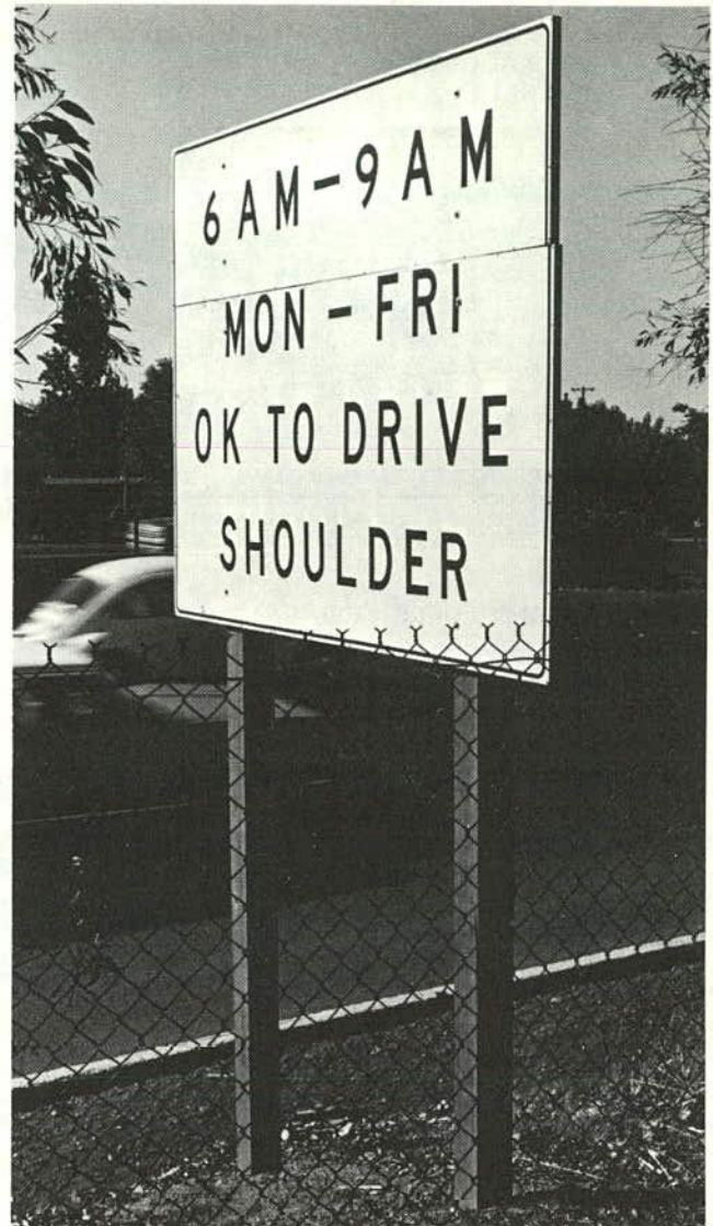
Figure 9. Signing for peak hour use of shoulder as a travel lane (California).
