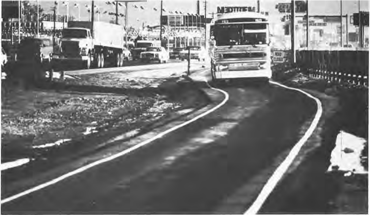
FIGURE 9 A connector lane provides continuity between concurrent flow and contraflow segments of exclusive bus lane. (Courtesy of American Public Transit Association.)
