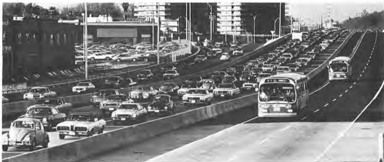
FIGURE 2 Shirley Highway (I-95) HOV express lanes in Washington, D.C. (middle lanes are reserved exclusively for buses and carpools).
