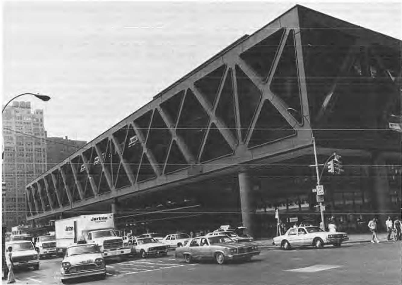
FIGURE 1 The Port Authority Bus Terminal in midtown Manhattan is an example of a level 5 transfer facility. It occupies one and a half square blocks, houses five separate bus loading areas on three different building levels, and has direct grade separated access to the Lincoln Tunnel. (Photo courtesy Port Authority of New York and New Jersey.)
