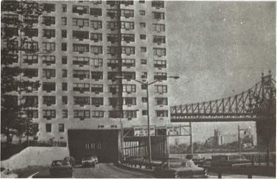
Figure 6. Sutton Place Apartments, over Franklin D. Roosevelt Drive, New York City. (October 1966 photo by Real Estate Research Corp.)
