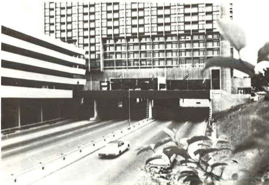
Figure 4. Gateway Center, over Massachusetts Turnpike in Newton, Mass. (June 1971 photo by Marshall and Stevens, Inc.)
