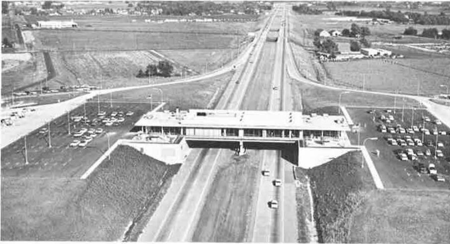
The Illinois Tollway Commission has built five over-the-roadway restaurants which allow a considerable reduction in land requirements as opposed to other types of road user service plazas. Shown here is the Des Plaines Oasis on the North-West Tollway. (Source: NCHRP Report 53.)
