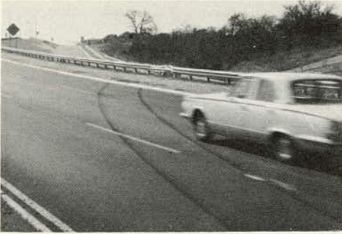
Figure 11. Skid marks indicate that curb caused vehicle to hit top of rail and roll down embankment.
