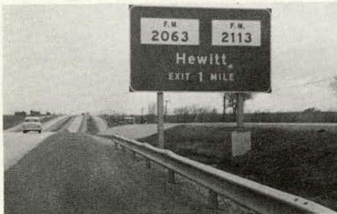
Figure 10. Flex-beam guardrail contains and redirects vehicle or, if straddled, stops the vehicle.
