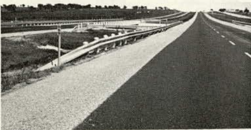
Figure 14. Example of a well-designed guardrail installation.
