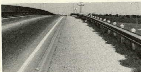
Figure 23. Guardrail transition at narrow bridge.
