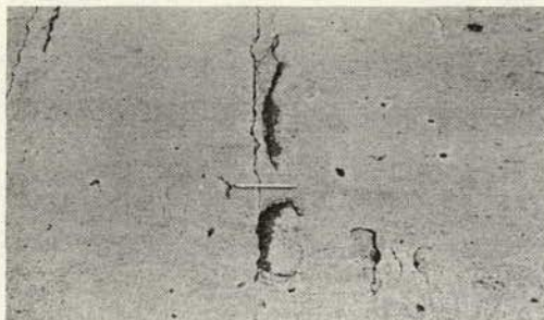
Figure 1. Typical surface spall associated with reinforcing steel.
