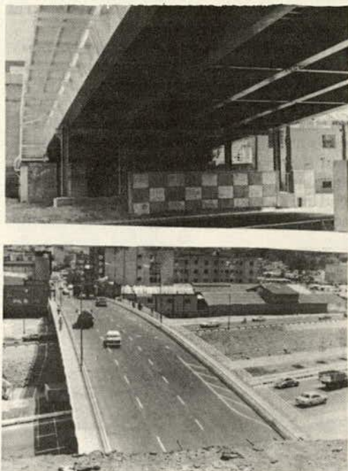
Figure 6. Fast-assembly bridge in Caracas.
